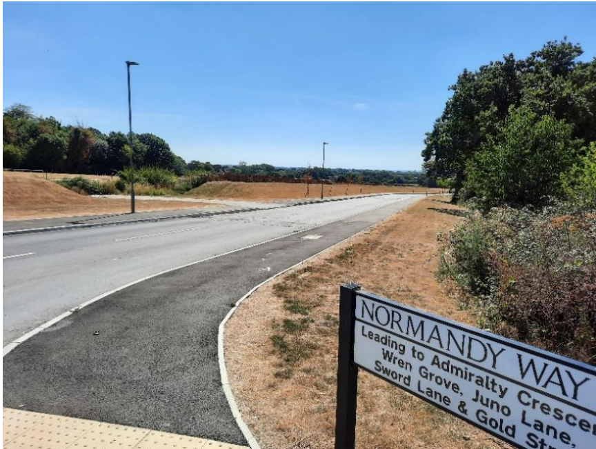
Photograph 2.2: Normandy Way looking south from Bartons Road towards the proposed site
