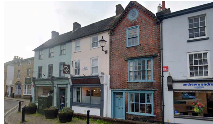
contrasting textures and tones to building frontages - dark textured/patterned brick and flint alongside smooth light render
