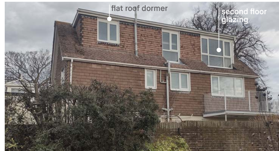
A - 72 Warblington Rd (view from within application site)
