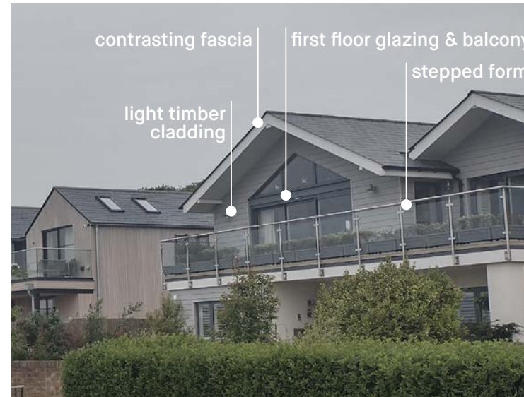
B - 9 Western Parade - contemporary replacement dwelling
