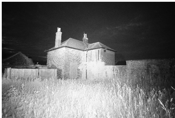
Photograph 3: A view from the camera located with the surveyor to the south-west of the building. Screenshot taken at the darkest point of the survey.
