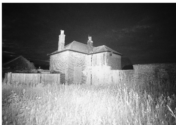
Photograph 1: A view from the camera located with the surveyor to the south-west of the building. Screenshot taken at the darkest point of the survey.
