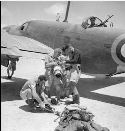
A Maryland Mk.I in North Africa, the Vickers 'K' dorsal position is clearly visible.
