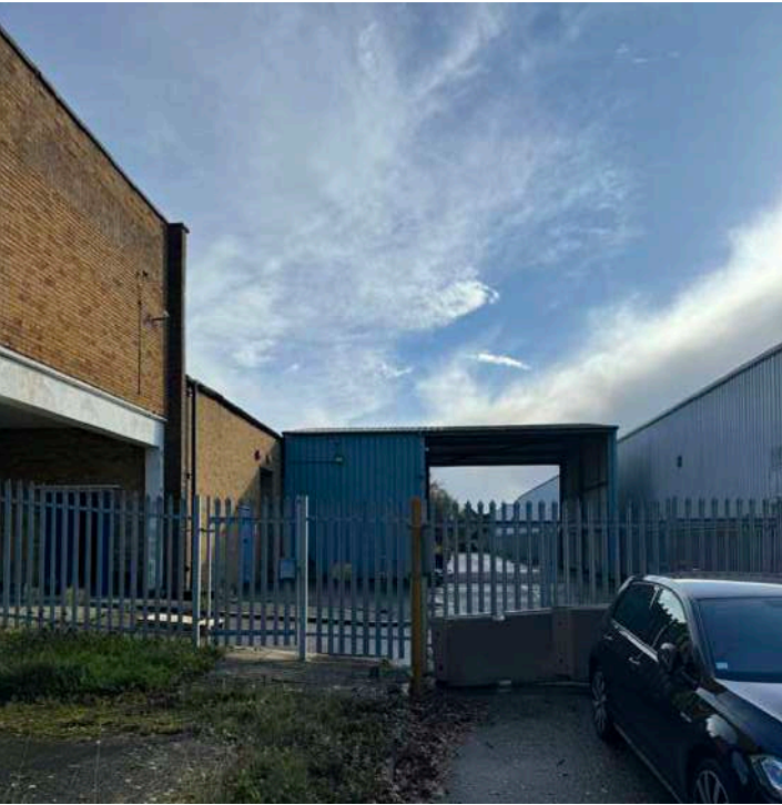
D Existing site entrance approach from south
