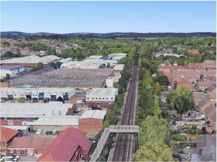
Aerial view looking North along Railway line separating commercial developments from residential developments along Proposed site Eastern boundary(rear)
