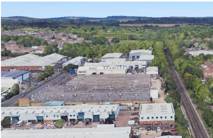
View towards northern boundary along railway line
