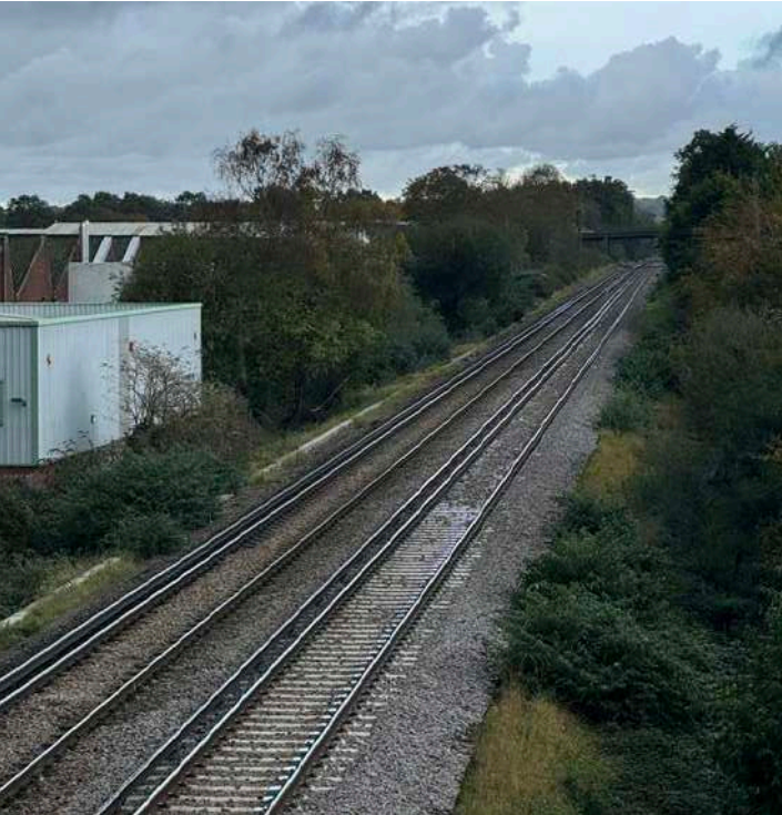
A View towards north along railway line
