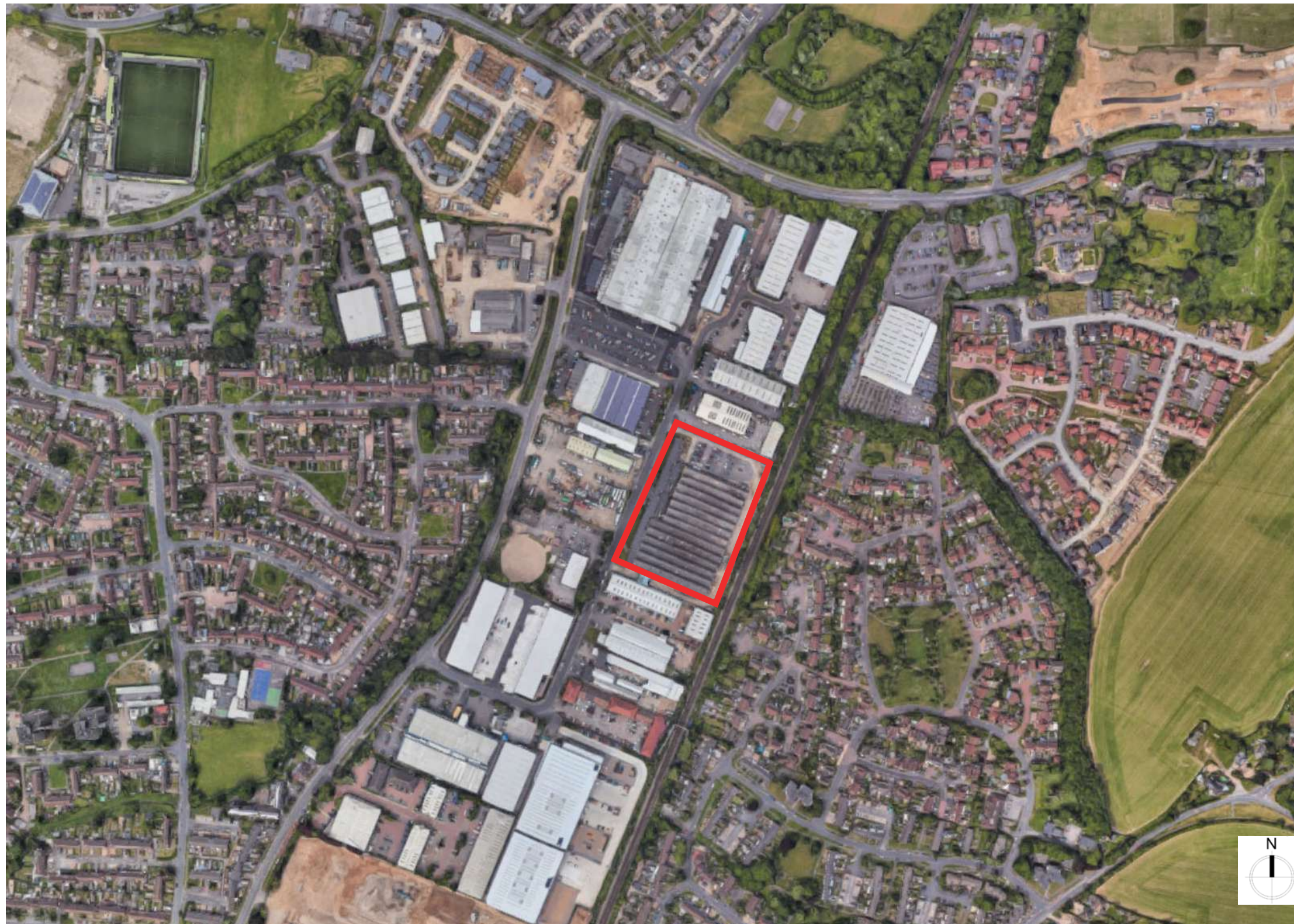
Aerial view of site towards North
