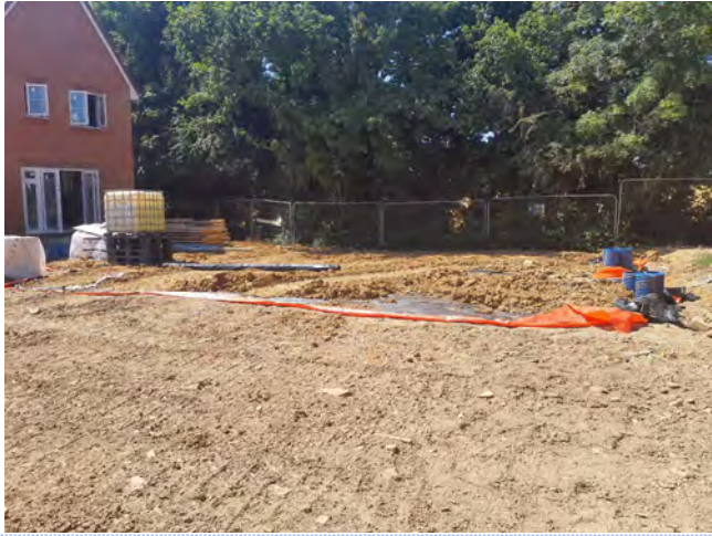
Description Plot 145 in progress
