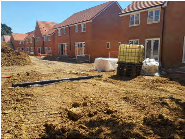
Description Plots 145-148 in progress
