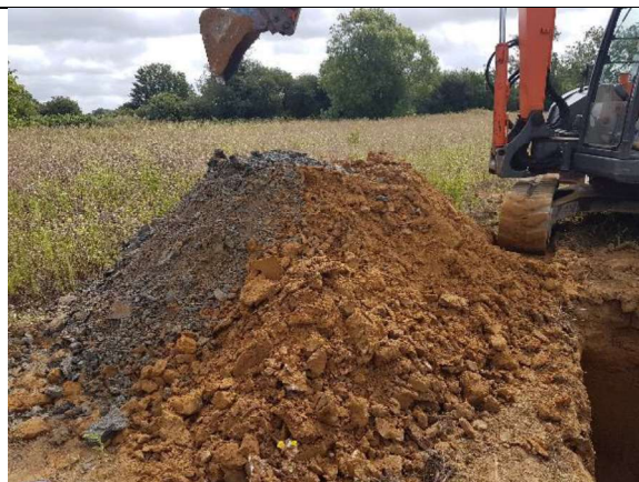
Plate 2 – TP01 – Trial pit spoil
