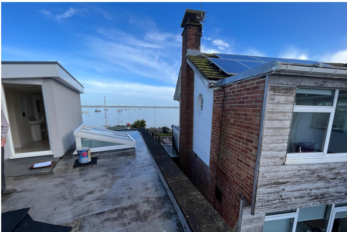
Figure 4 View Looking North between Small First Floor Addition & Sinah House
