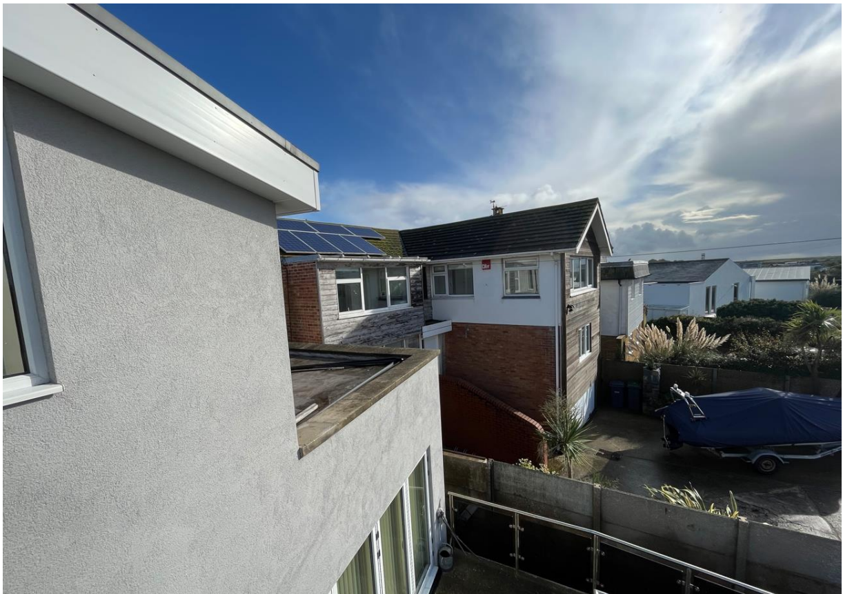
Figure 8 View from Front First floor Balcony towards front of Sinah House
