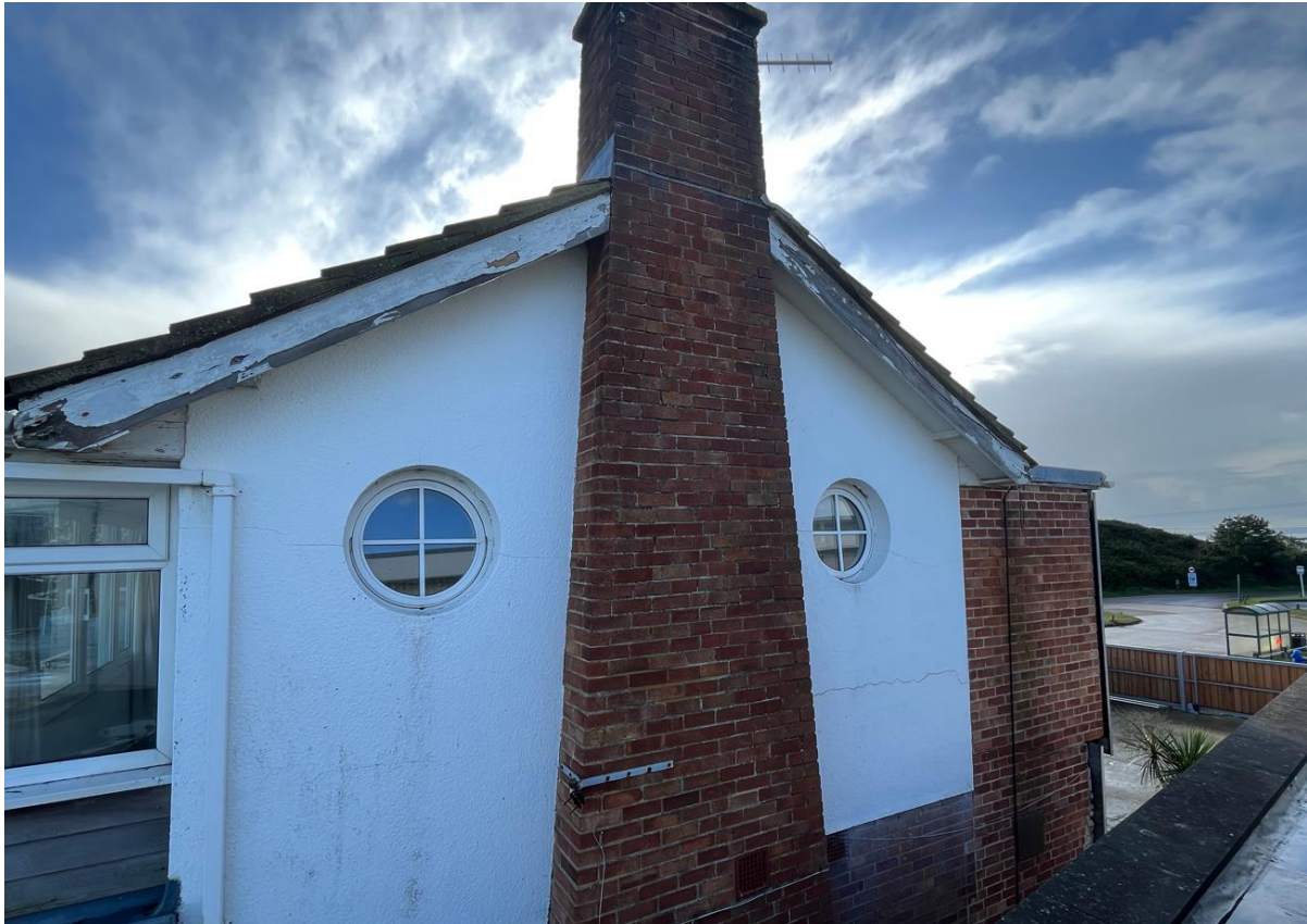
Figure 5 View of West, First Floor, Elevation of Sinah House
