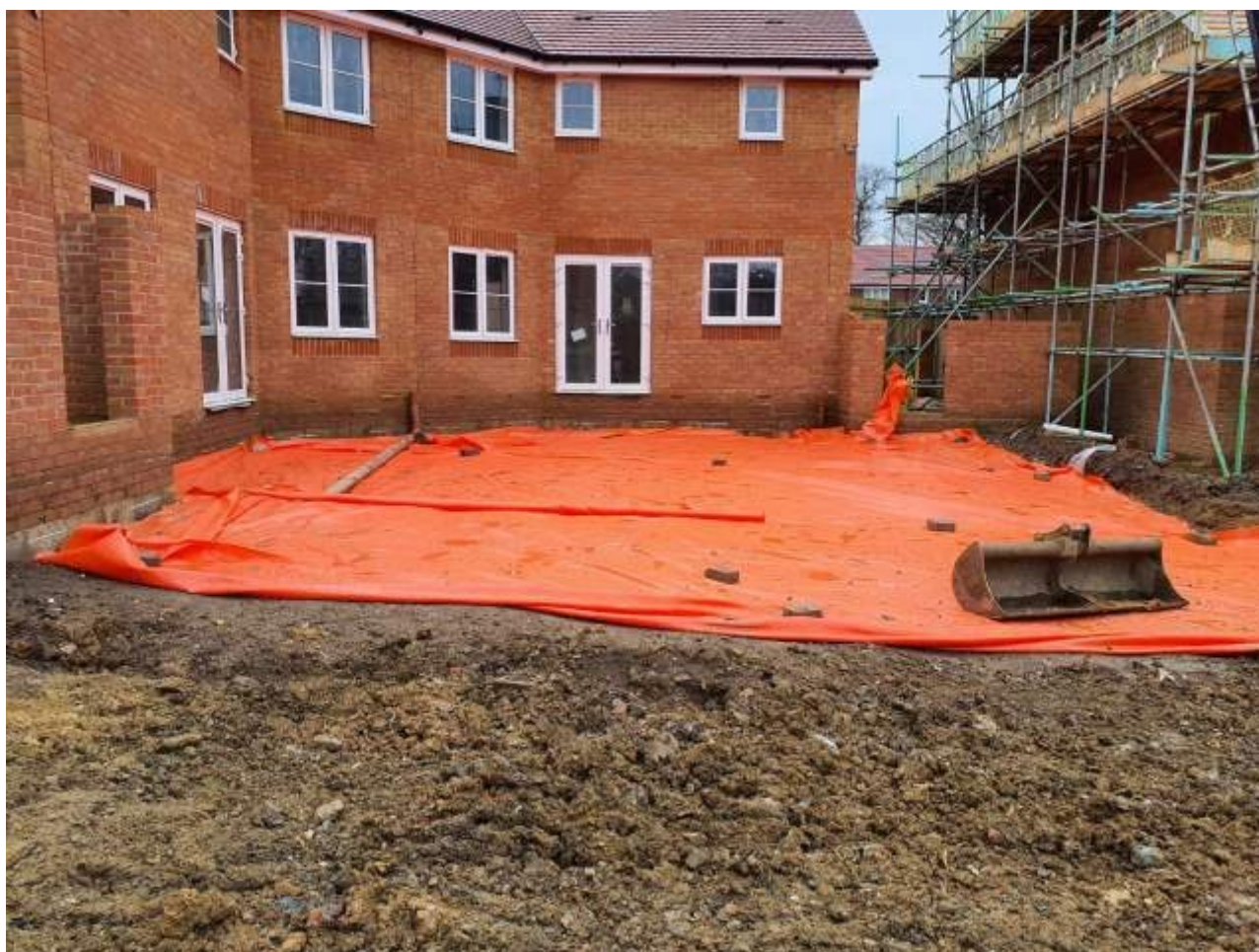
Plate 4 – Orange geotextile laid across plots
