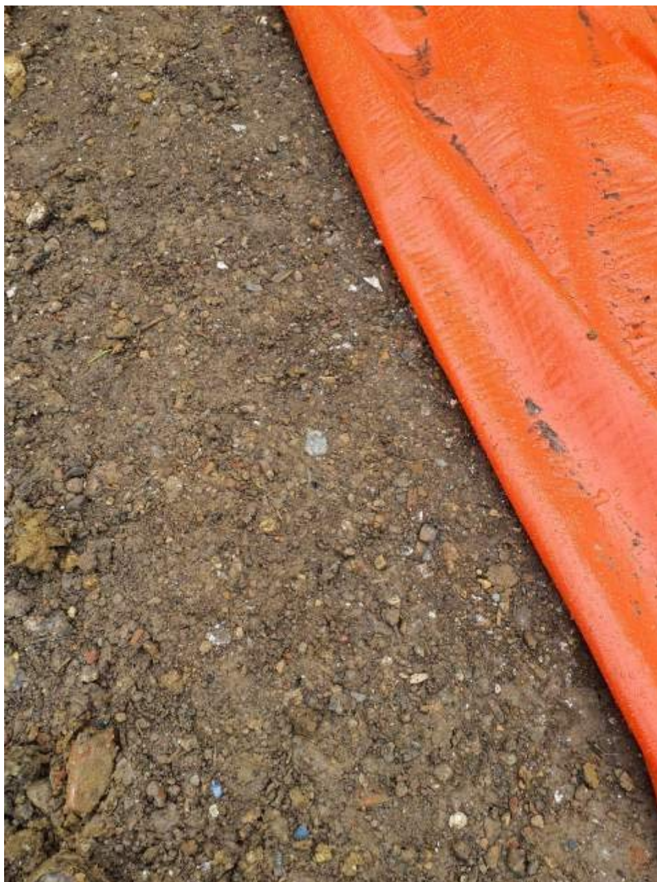
Plate 3 – Orange membrane rolled back to reveal crushed layer
