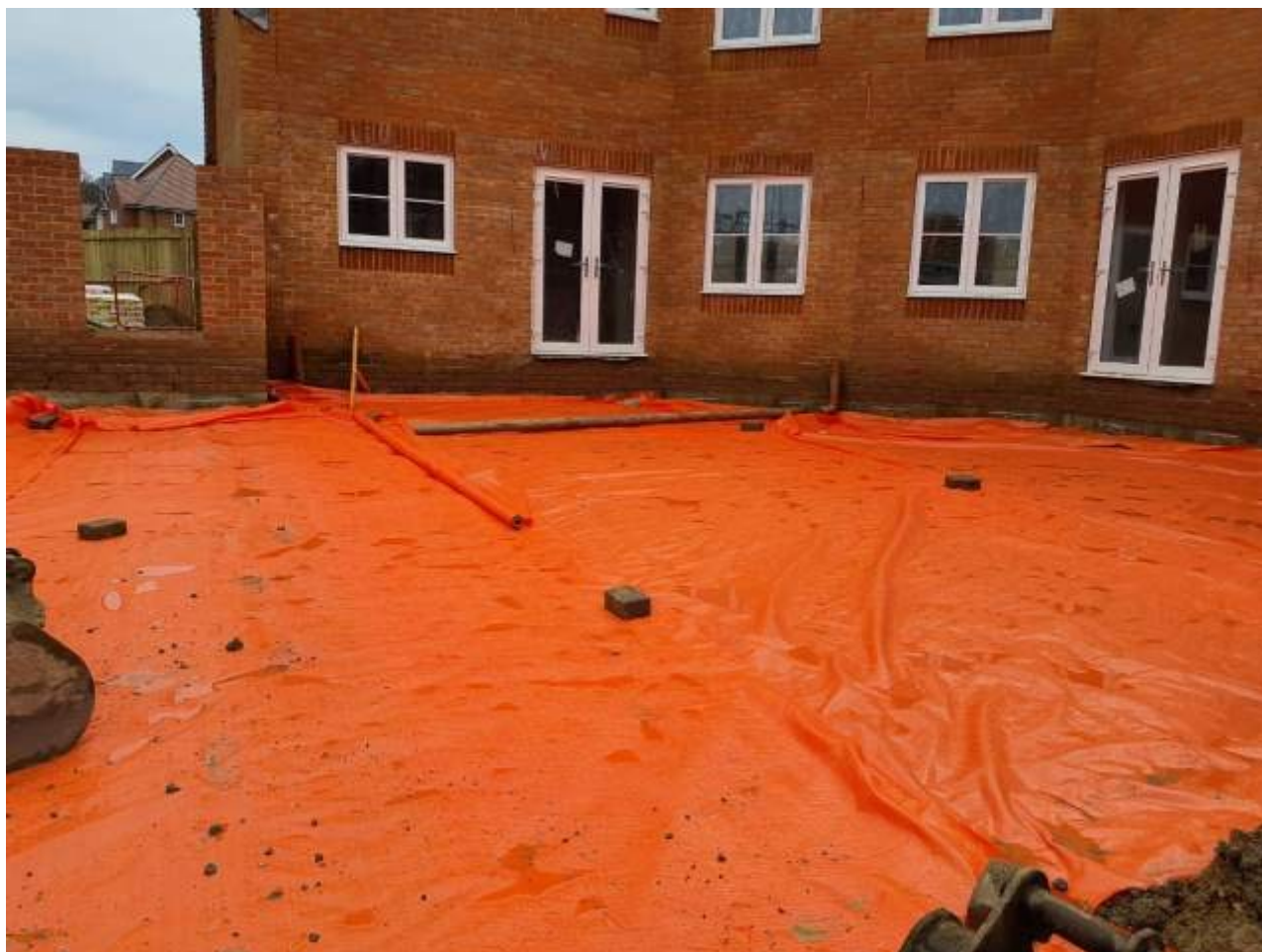
Plate 2 – Orange geotextile laid over crushed concrete layer on Plot 124
