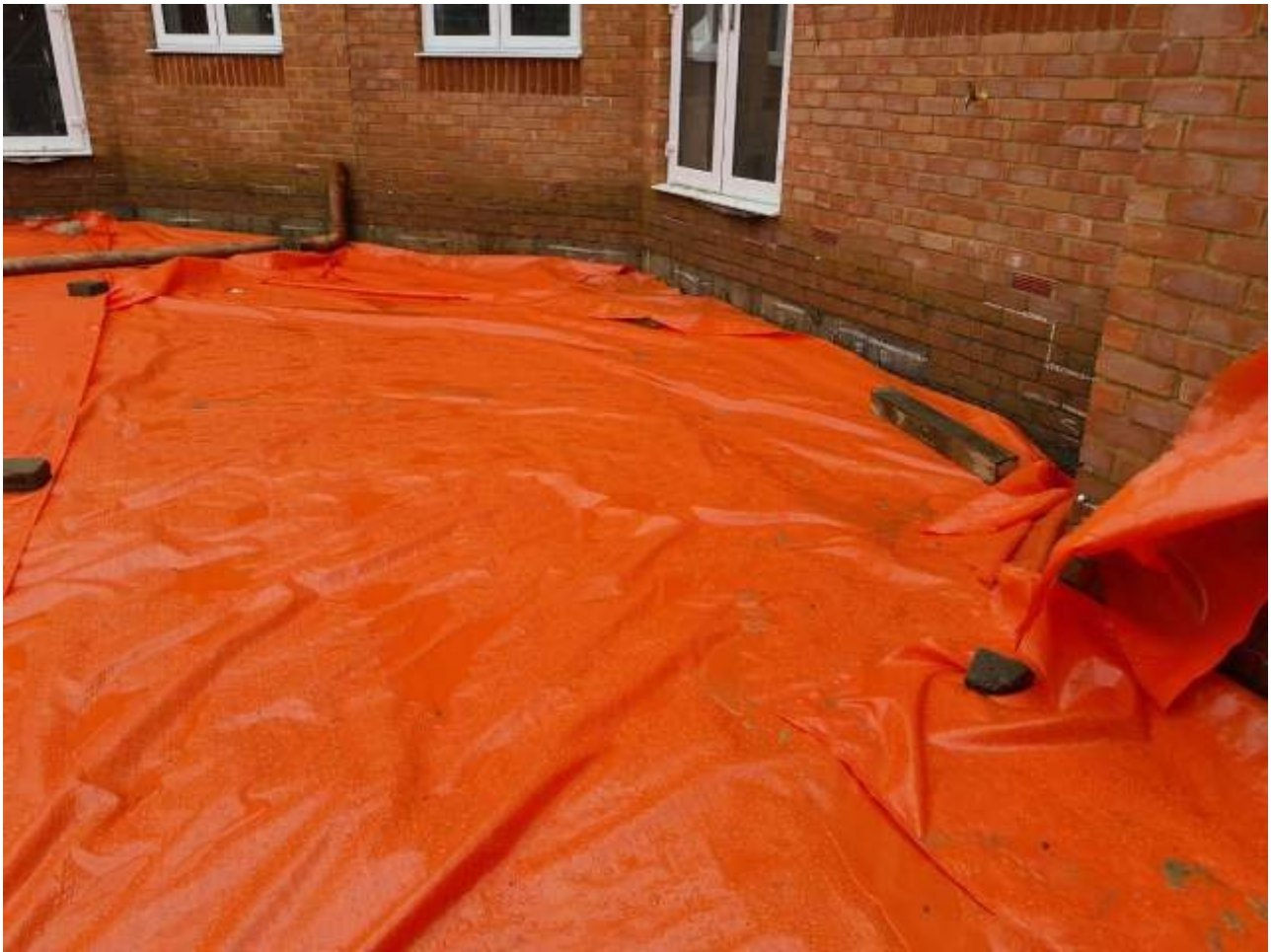
Plate 1 – Orange geotextile laid over crushed concrete layer on Plot 123
