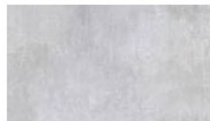
smooth concrete finish to horizontal planes
