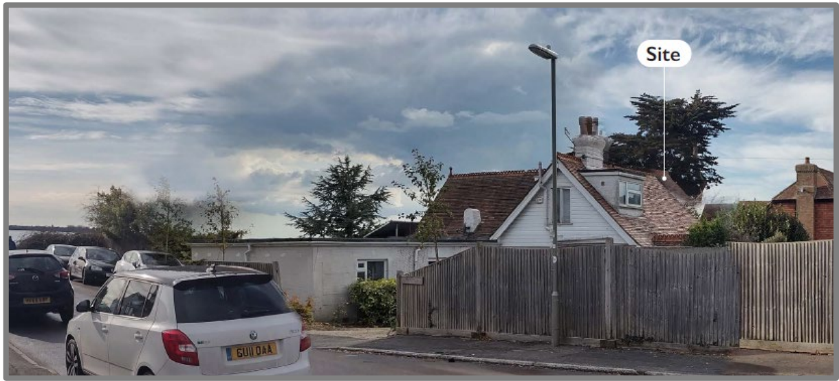
Figure 1: Photograph of existing dilapidated dwelling taken from OB Architecture's DAS
