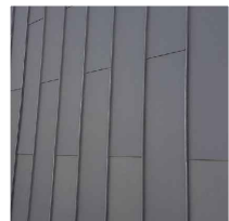
2. VMZINC STANDING SEAM CLADDING ANTHRACITE GREY SEAMS AT 400mm CTRS
