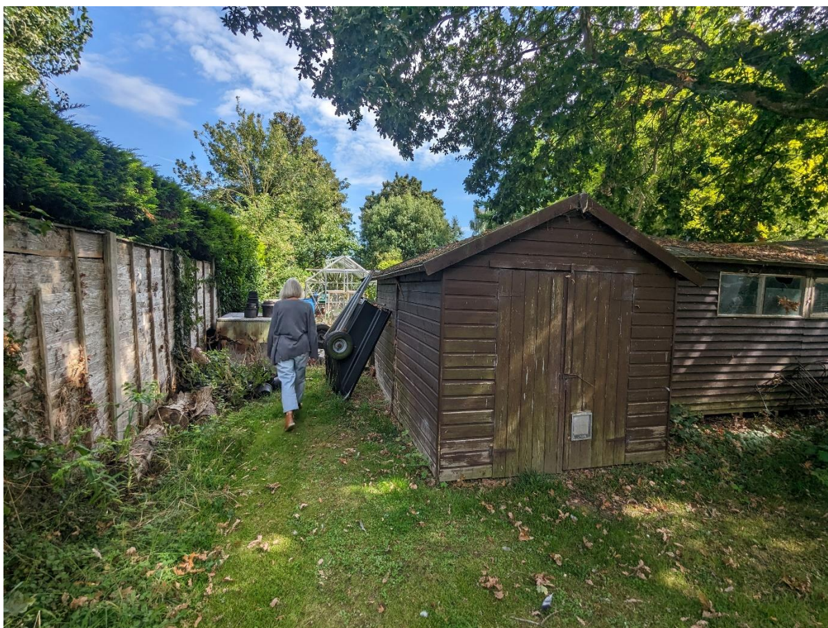
Fig 8 Shed and greenhouse to be removed to allow for access to the new dwelling
