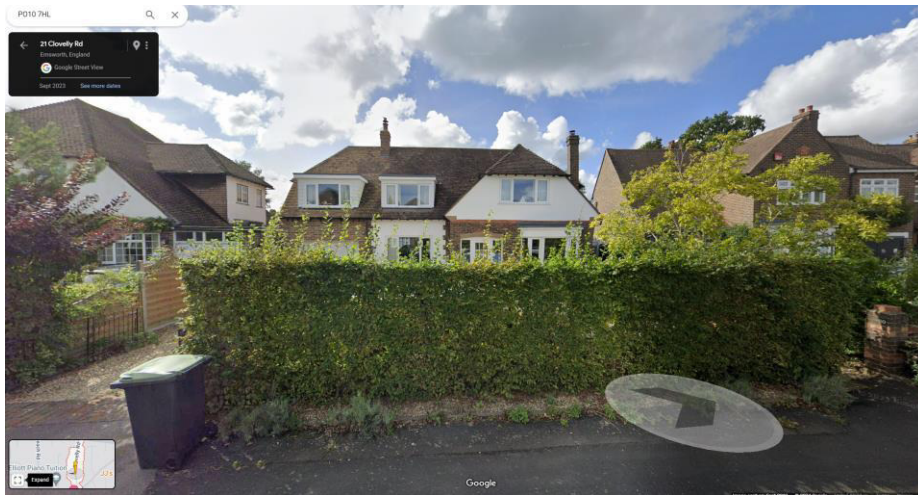
Photograph 1 – East elevation Image from Google
