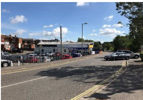
View looking north on Rockville Drive
