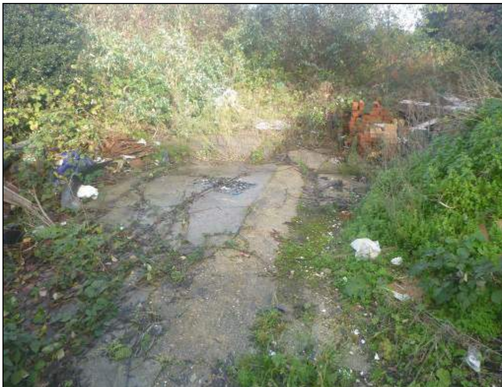
Photograph 3 Showing the ground surface at the site
