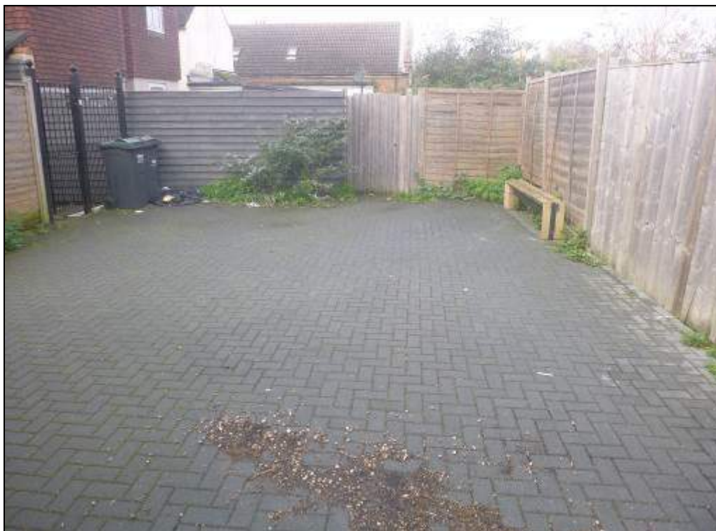
Photograph 2 Showing the block paved area at the rear of the dwellings
