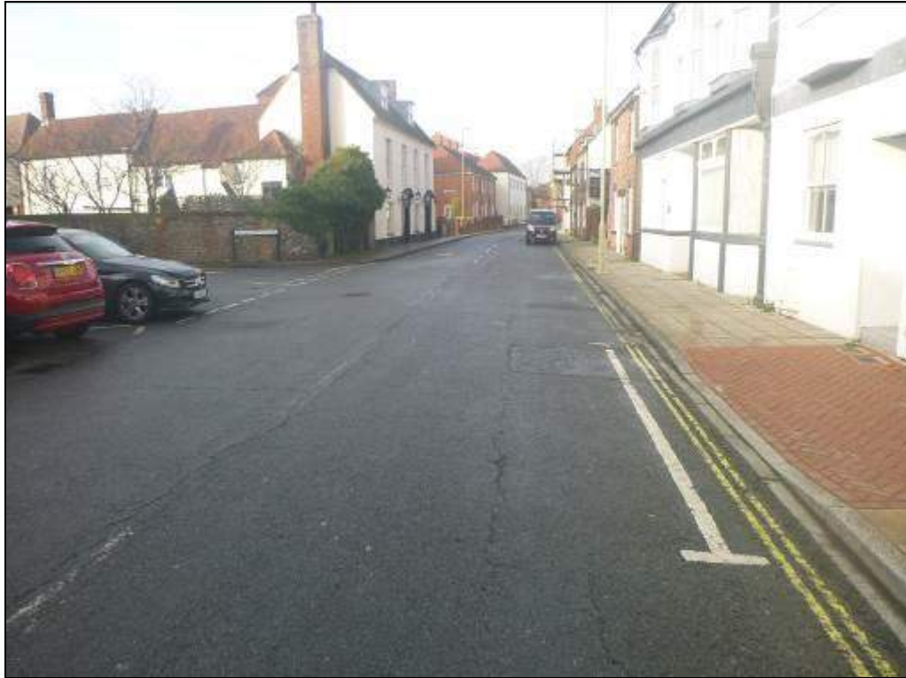
Photograph 6 Showing West Street looking northwestwards
