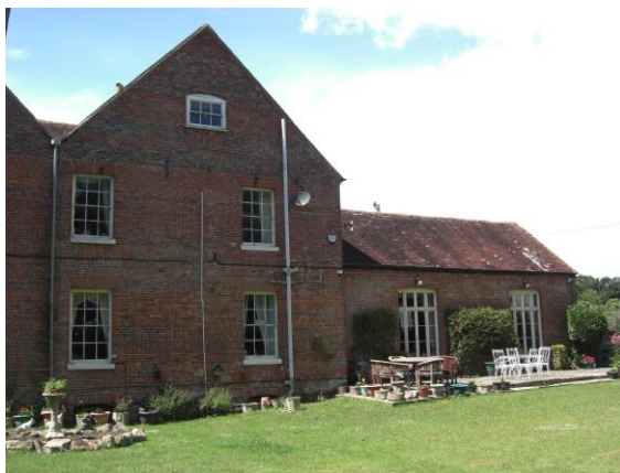
Part east elevation with lower north range
