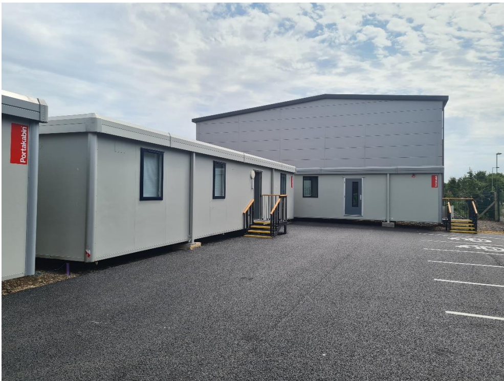
Figure 08 - Portakabins in situ
