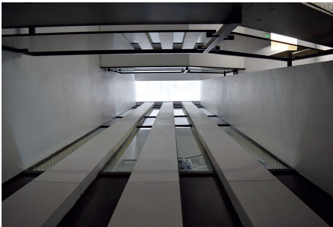
Plate 168: South part of Building 6000, staircase skylight.
