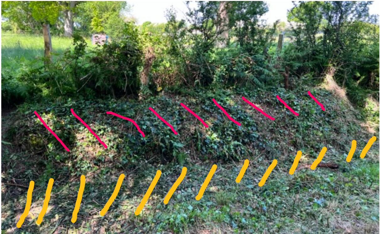
Photo 5: The depression that requires infill is hatched yellow. The extent of earth bank that requires removal is hatched red.
