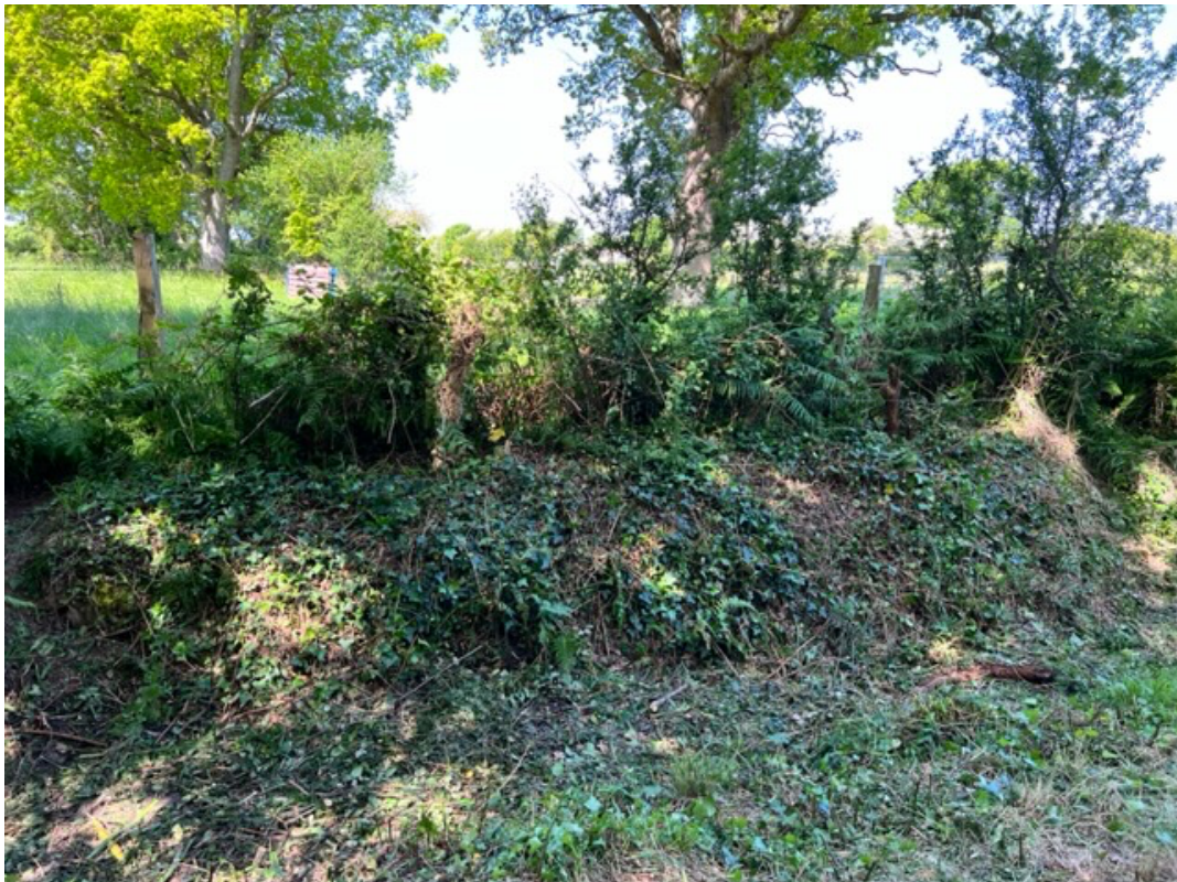
Photo 1: Looking west at the depression and small earth bank. The new alternative access lies in the field owned by Mr & Mrs Phillips behind.
