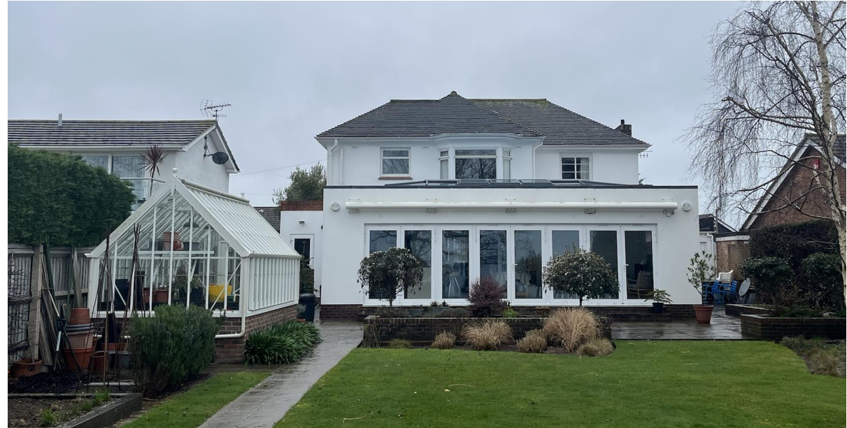
View of existing dwelling from the rear garden.
