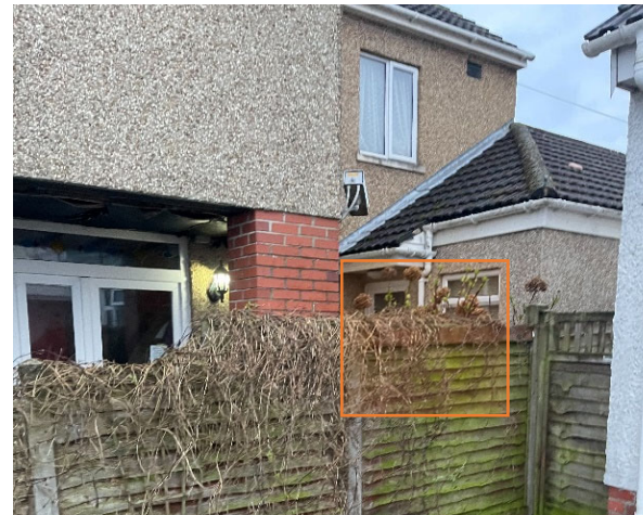
Figure 5.1 – Location of windows in 6 Privett Road
