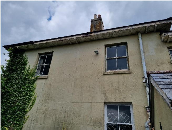
Photo 5: East facing elevation
