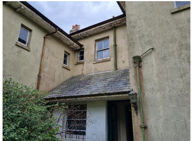
Photo 8: North facing porch
