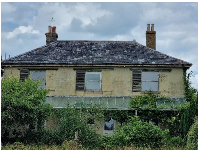
Photo 3: South facing elevation
