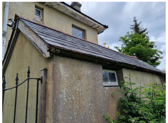
Photo 4: East facing elevation
