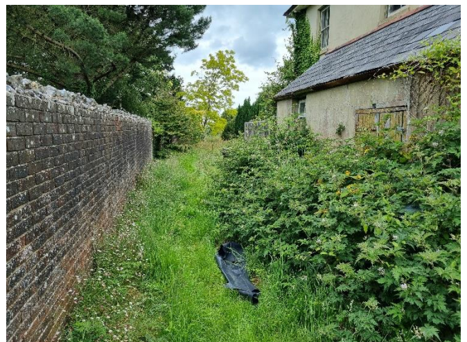
Photo 10: Side passage looking south
