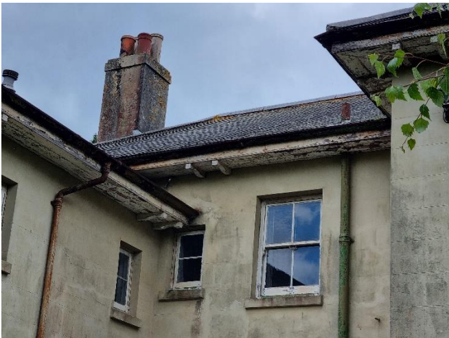
Photo 7: North facing elevation
