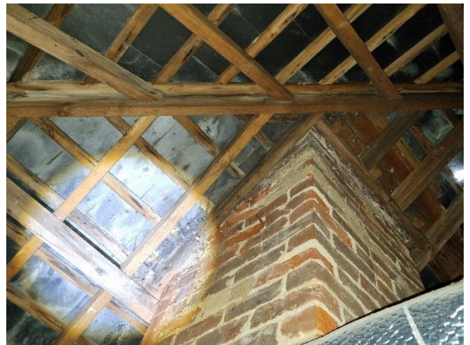
Photo 2: Interior loft void
