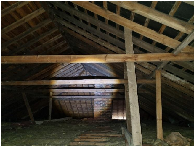
Photo 1: Interior loft void
