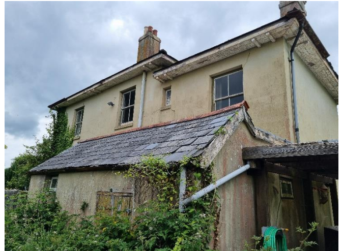
Photo 6: East facing elevation
