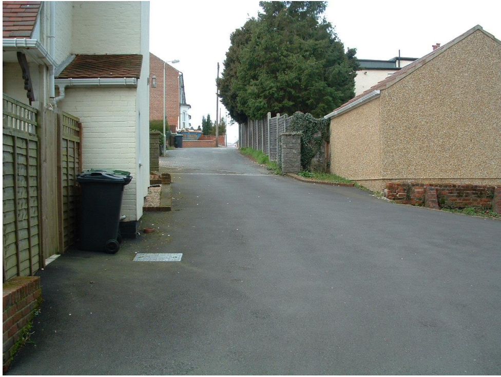
View of existing access road
