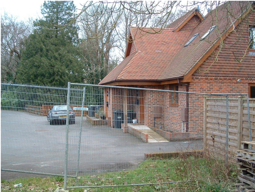
View of adjoining properties of No.34 and No.36
