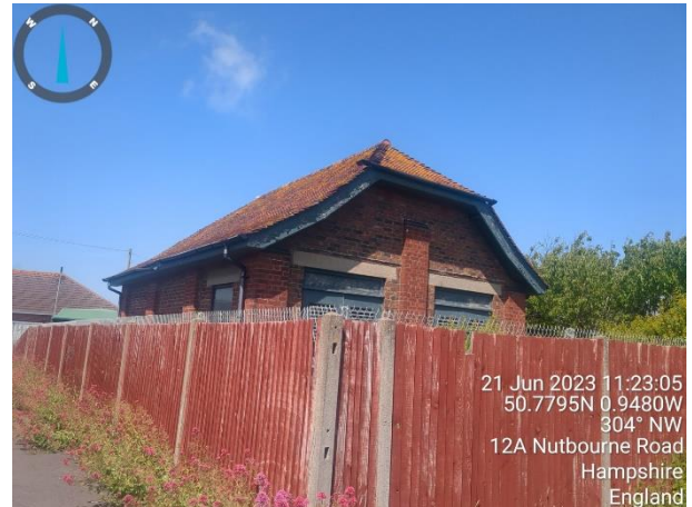
Photograph 8: View of the rear and southern side of building.
