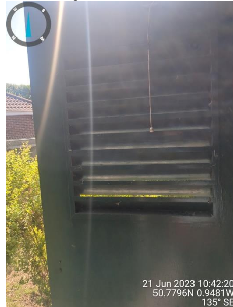
Photograph 16: Close up of the vents on the doors that are the only entry/egress feature to the interior at the rear.
