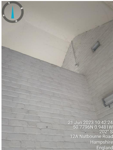
Photograph 17: View of the interior from the rear half of the building, separated by wall in the middle but open to the roof.
