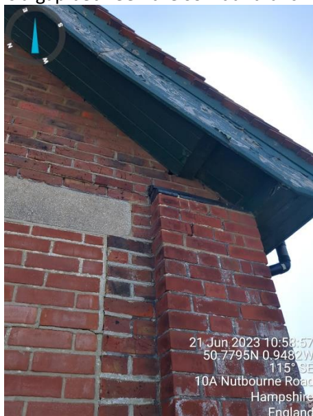
Photograph 9: View of the rear soffit where there is a gap between the soffit and brickwork.
