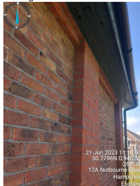
Photograph 6: View of soffit that extends along the south and north elevations which is flush with the brickwork.
