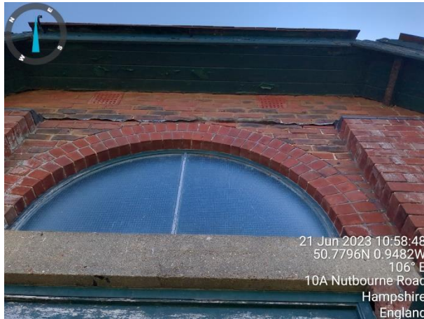
Photograph 7: View of the front of the building with a gap present between brickwork and soffit and gaps in brickwork on top corner of doors.
