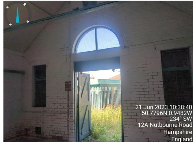
Photograph 14: View of the front door from inside the building.
