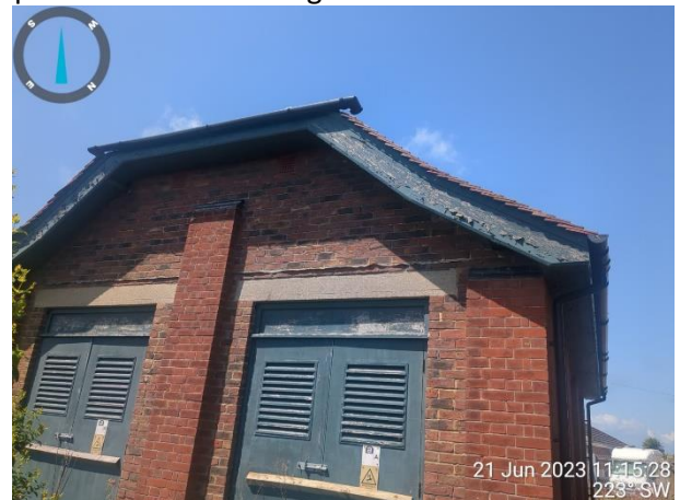
Photograph 4: View of rear of rear elevation of the building.
