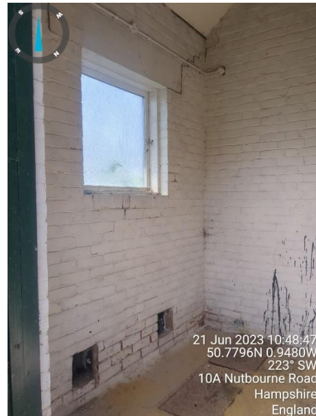
Photograph 18: View of the interior which is lit by a square window on either side.
