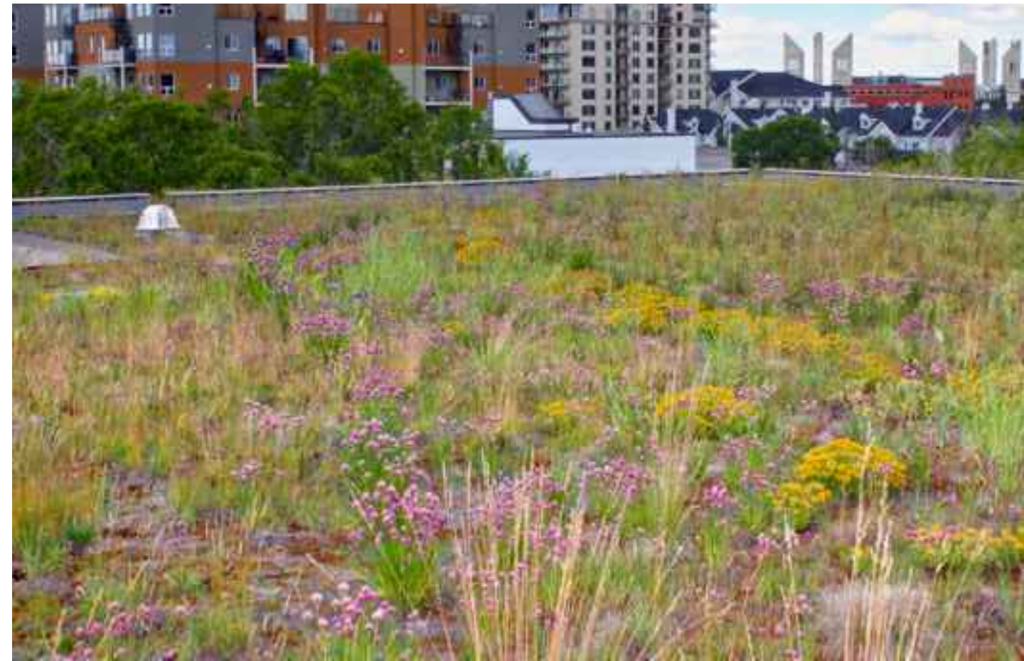
C. Green Roof
