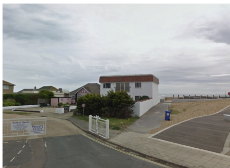
Existing Exposed View
