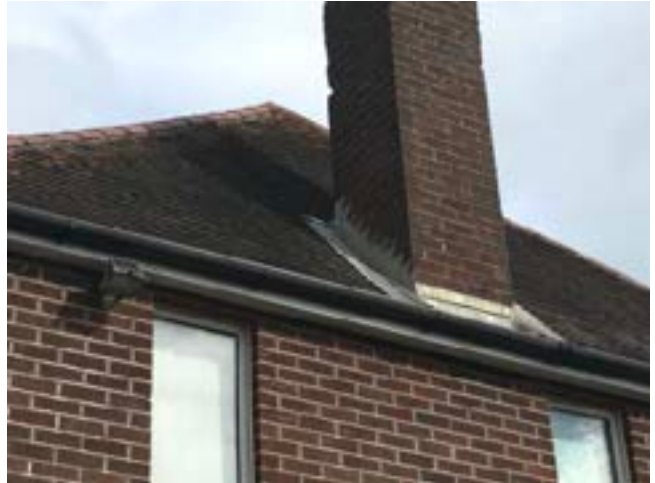
Image 10: View of the southern hip with tight lead flashing around the chimney and intact ridge and roof tiles.
