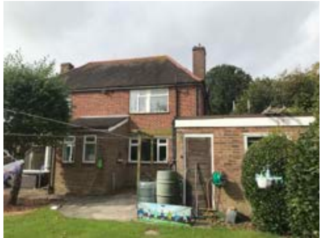
Image 12: View of the western elevation of the main dwelling and garage.
