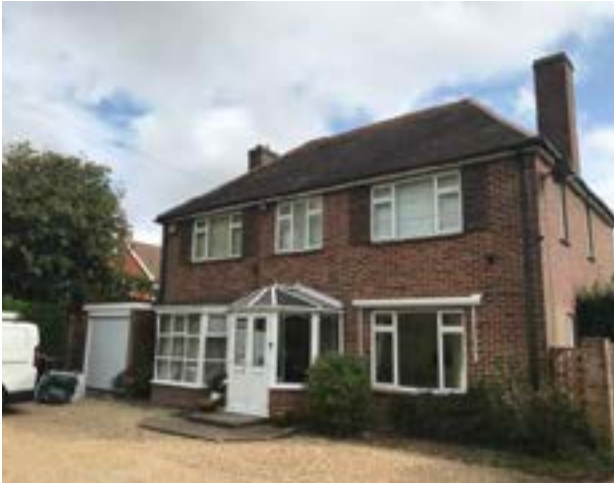
Image 9: View of the western elevation of the main dwelling and garage.
