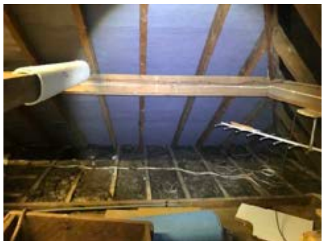
Image 14: Breathable membrane on the eastern pitch.
