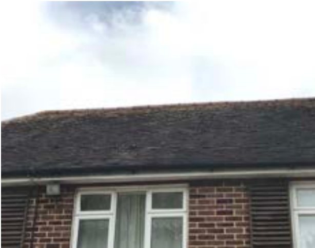
Image 11: Tight roof tiles on eastern elevation.
