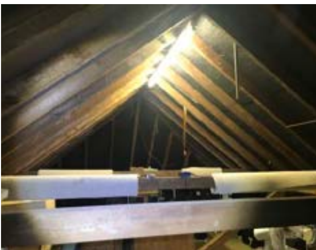
Image 13: View of the loft void.
