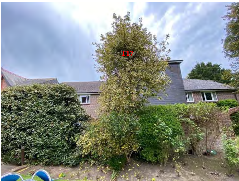
Photoview 15: View west at T17.
