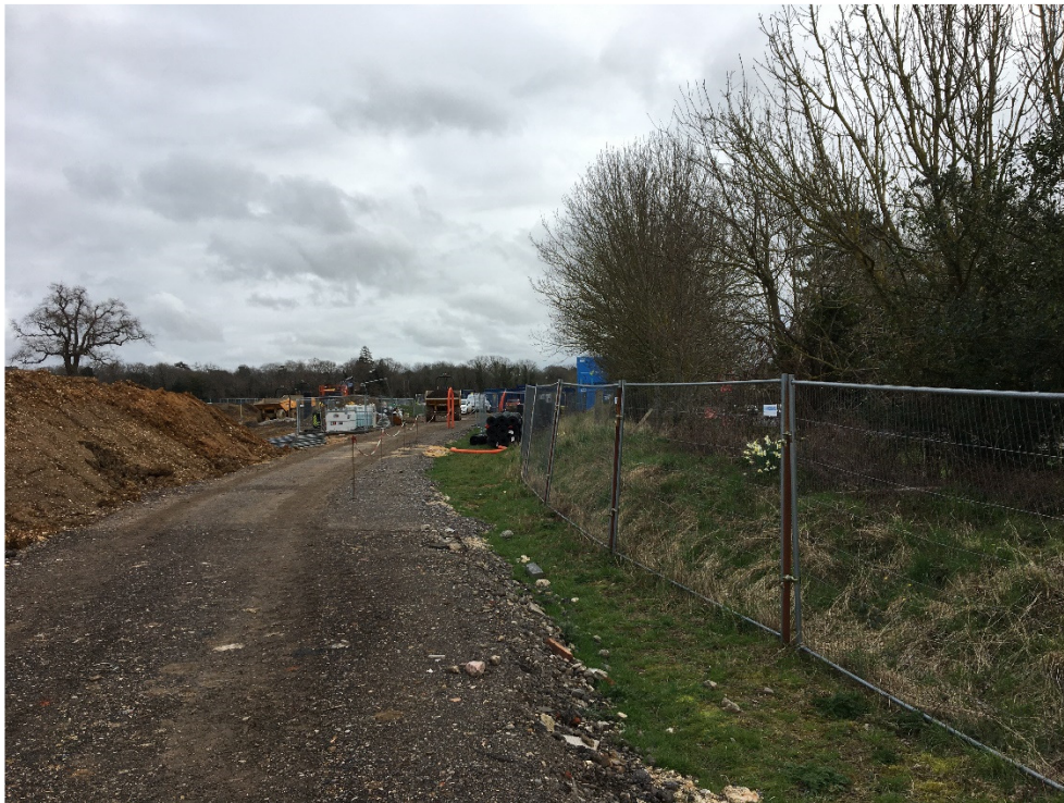
Figure 2. View looking eastwards. Bartons Rd to the right.
