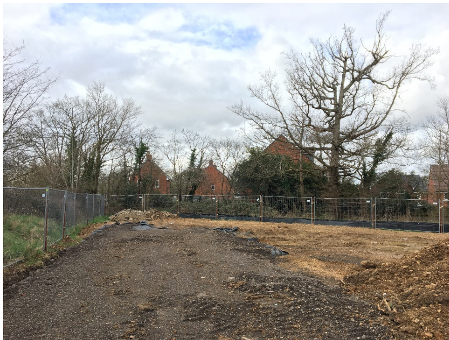
Figure 4. View looking westwards. T22 on the right side of the picture. Pilling mat in view.
