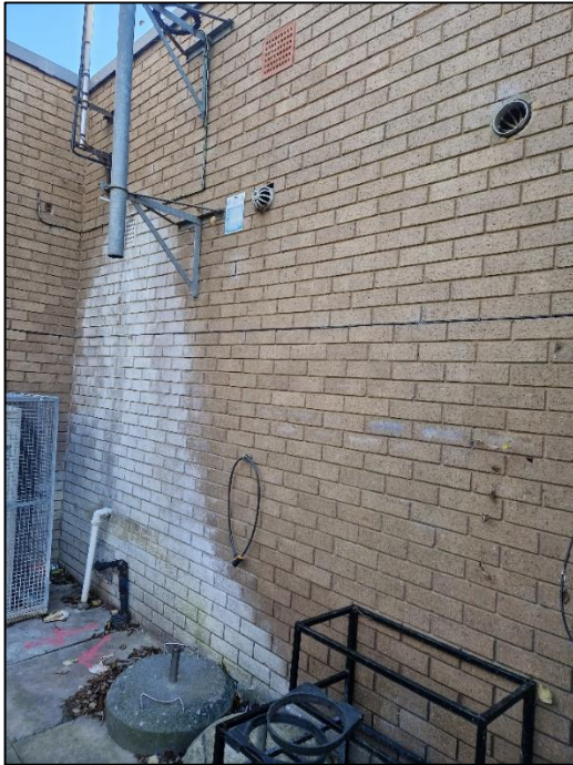
Photograph 6 showing the brickwork
