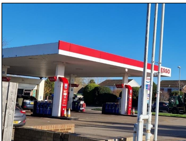
Photograph 5 showing the forecourt canopy
