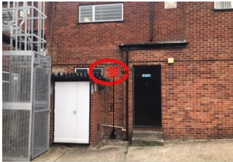
Side Elevation Photo
