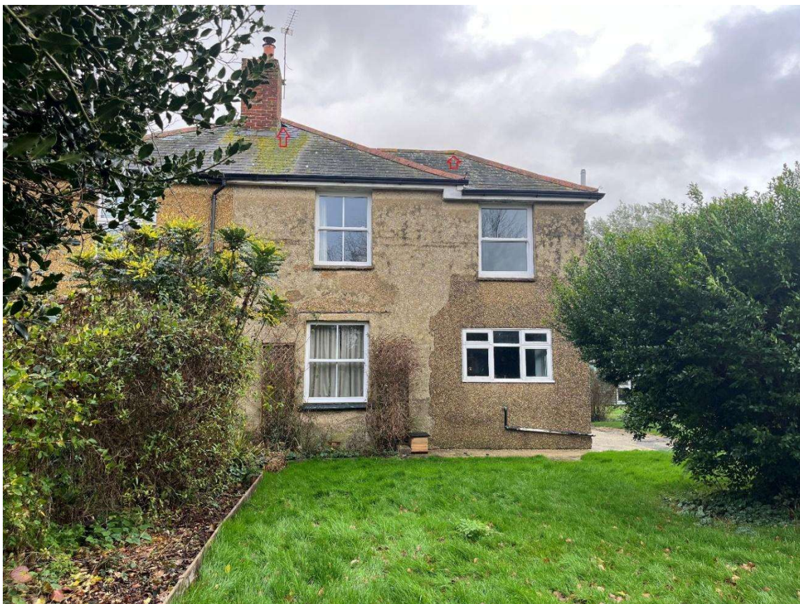
Figure 1. Western elevations looking east. Red arrows indicate potential access points for roosting bats.
