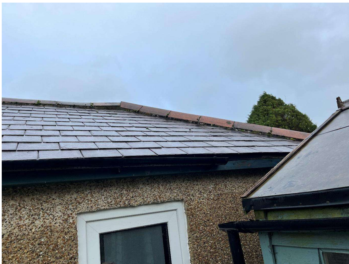
Figure 4. Garage roof looking east.
