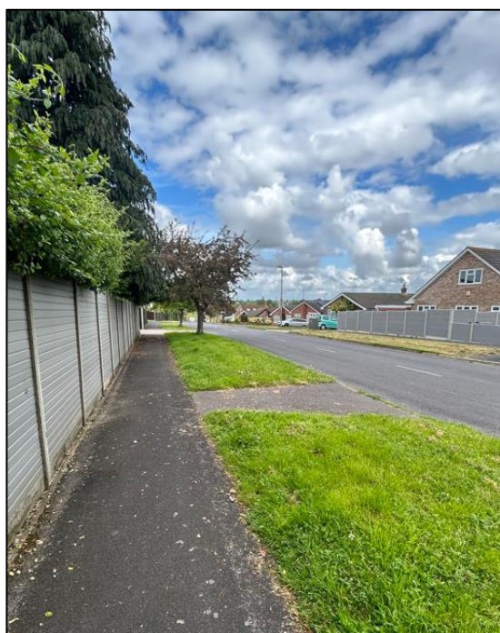
Photograph 25: Footways Along St. John's Avenue
