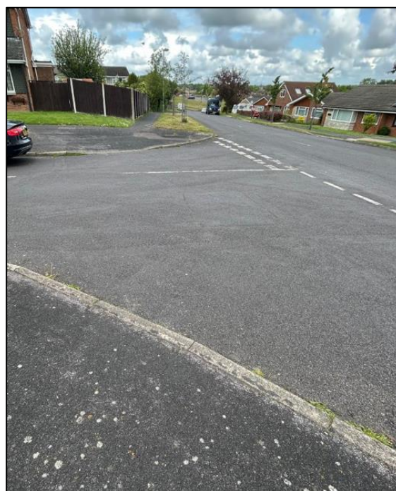
Photograph 26: Dropped Kerbs across Junctions along St. John's Avenue
