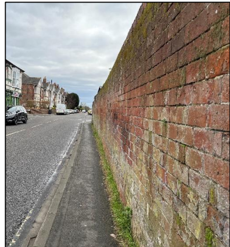
Photograph 45: Southern footway along West Street
