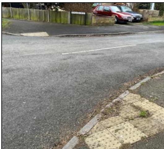
Photograph 40: Scratchface Lane/Maylands Road conditions
