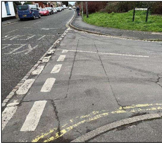
Photograph 44: Merywick Road/West Street junction
