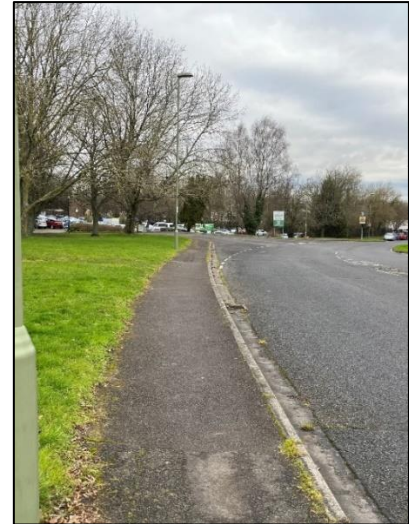
Photograph 35: Footway along western side of Crookhorn Lane
