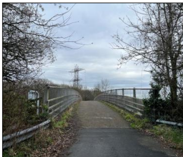
Photograph 38: A3(M) bridge crossing
