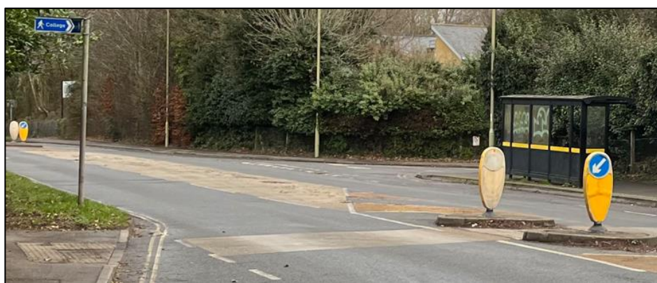
Photograph 9: Crossing point across College Road
