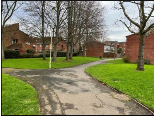
Photograph 10: Pedestrian infrastructure linking Atlantis Avenue to Crookhorn Lane
