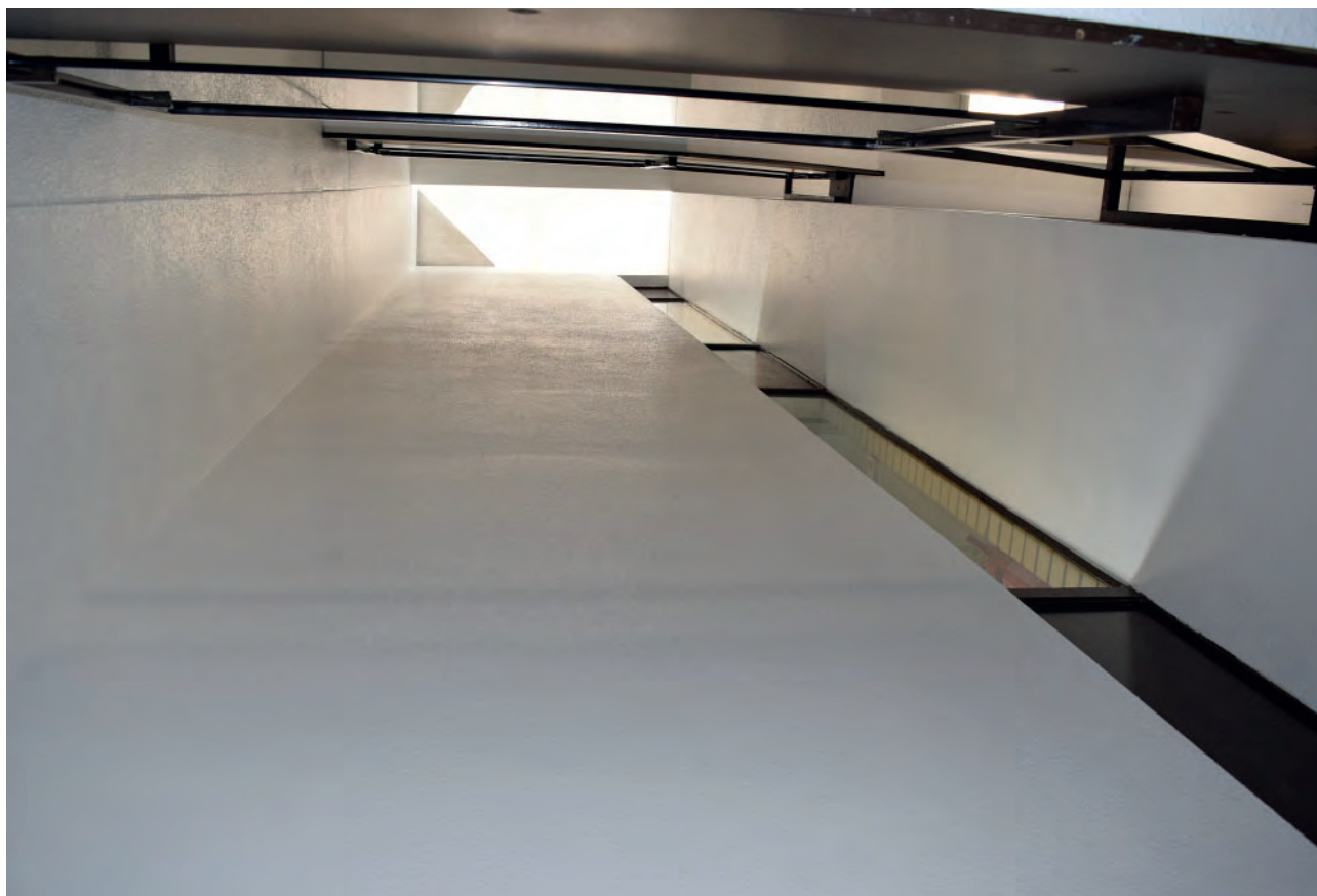
Plate 157: North part of Building 6000, staircase skylight.
