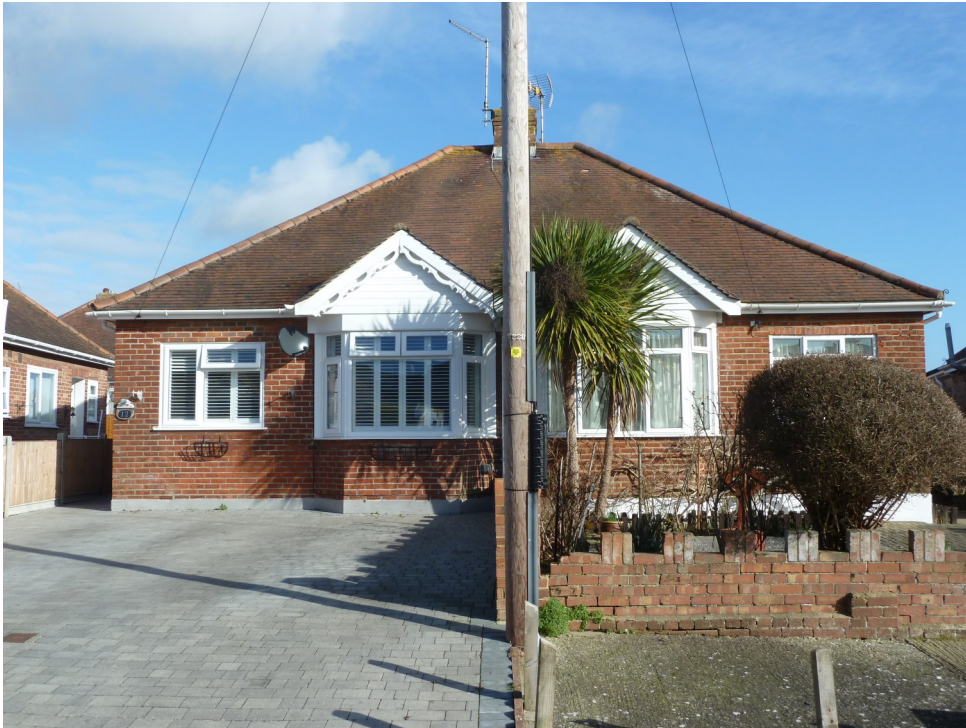
11 Typical pair of semi-detached bungalows on Ingledene Close.
