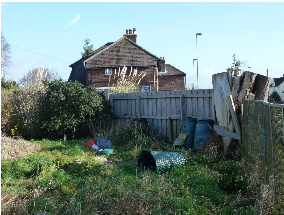
6 Part of the existing soft landscaping and temporary boundary fencing. Tree stump to be removed to allow for a continuous brick boundary wall.
