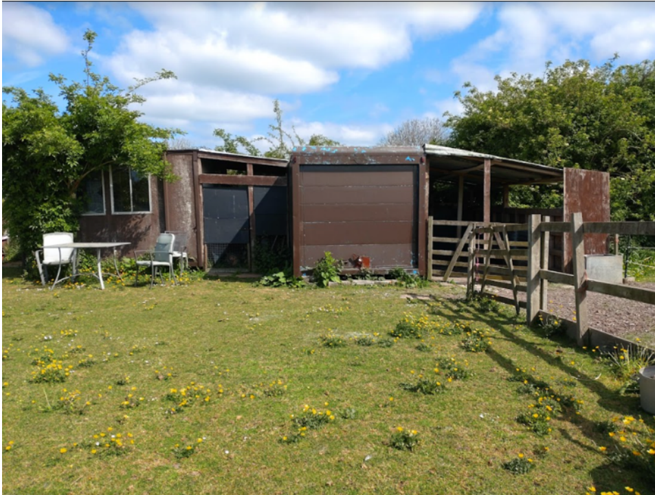
Figure 6. View of one of several horse stable/shelter structures present on-site (taken May, 2022).
