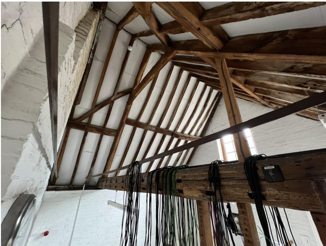
Photograph 4 – Roof rafters and Trusses at west end of building. Similar to arrangement shown on section A-A and B-B; although some adjustments in this area to make vaulted.
