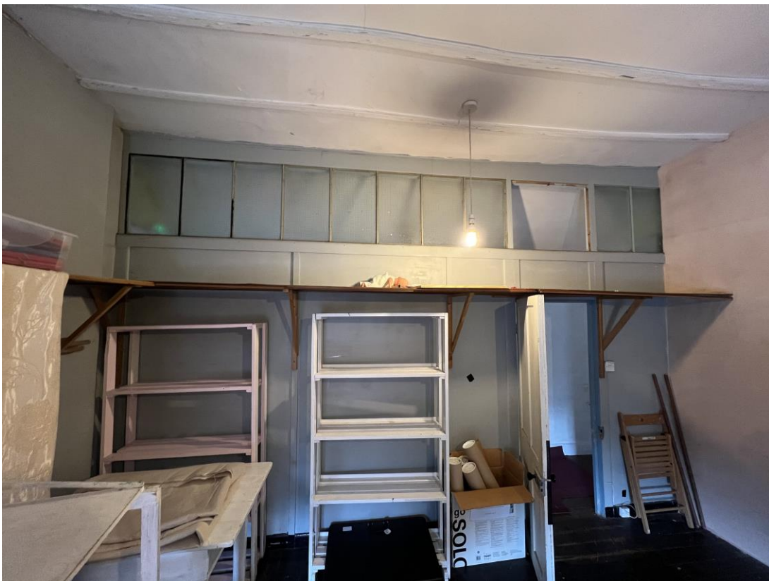
Photograph 2 – Partition to be removed at first floor
