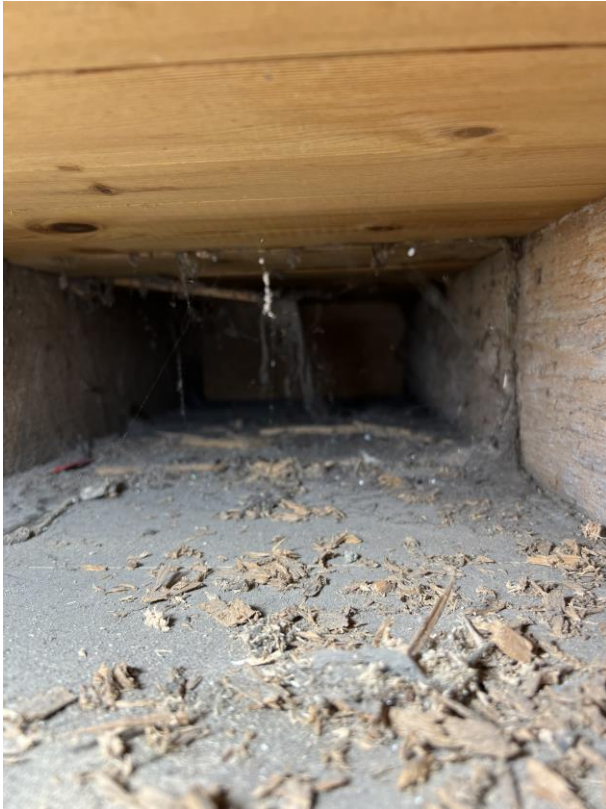
Photograph 3 – Ceiling void at first floor as shown on sections A-A and B-B
