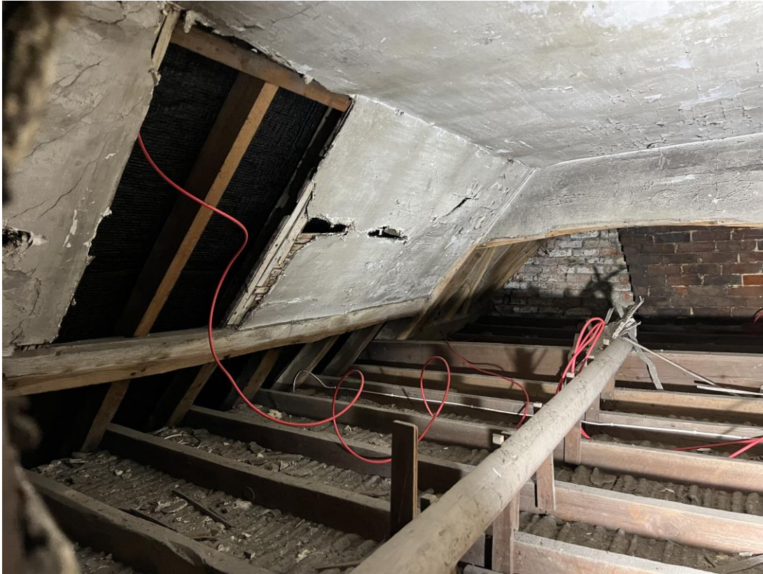
Photograph 1 – Roof void as shown on sections A-A and B-B
