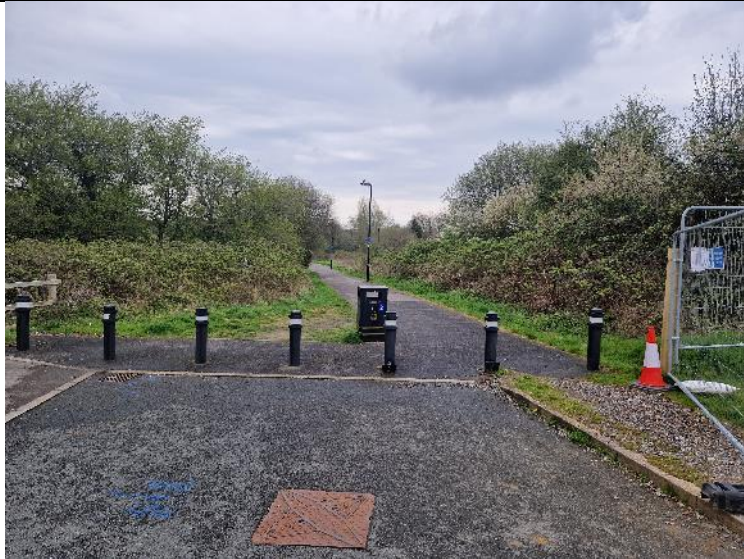
PLATE 01 – Site Entrance – Looking North.
