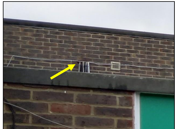
Photo 11 Hole for multiple cables on the NE elevation of room 60 (feature 3)
