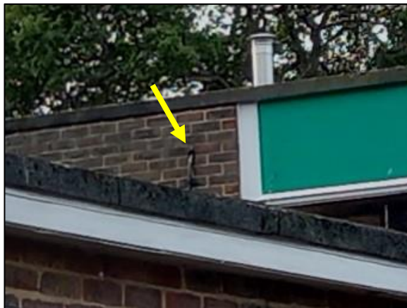
Photo 12 Hole for cable on the NE elevation of room 63 (feature 5)
