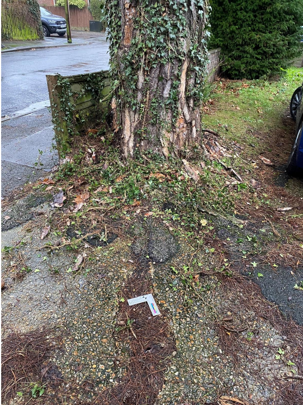
SAL4 T1 with direct damage to access driveway.
