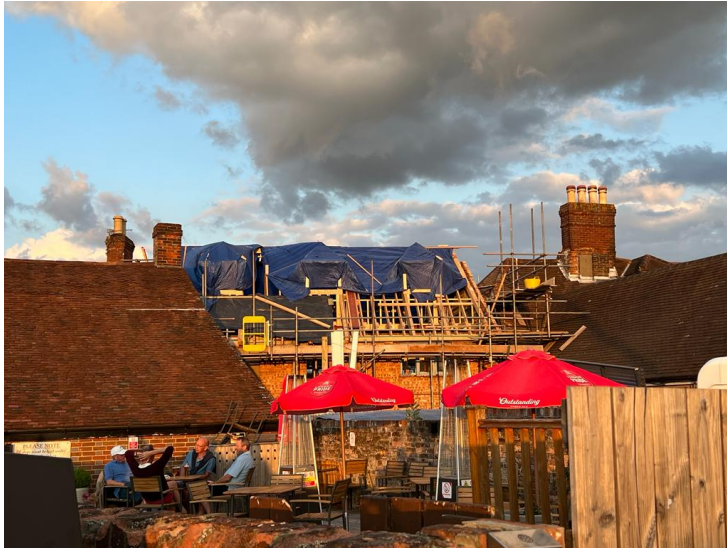
Multiple dormers being constructed on front façade
