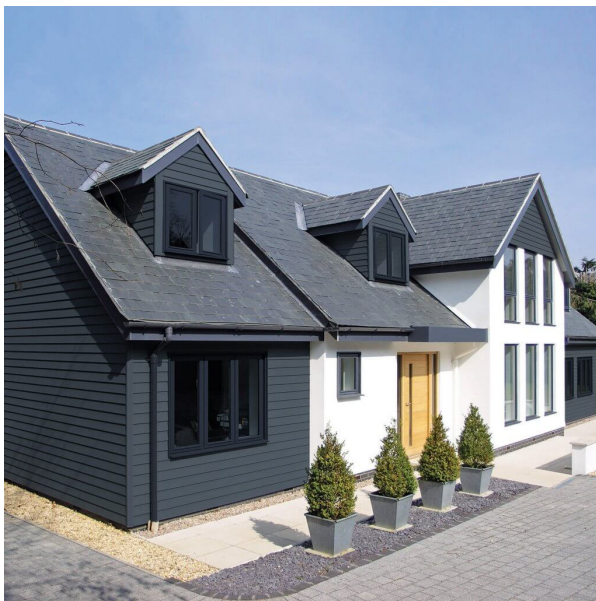
Combination of dark framed PPC aluminium windows & doors, render and composite cladding
