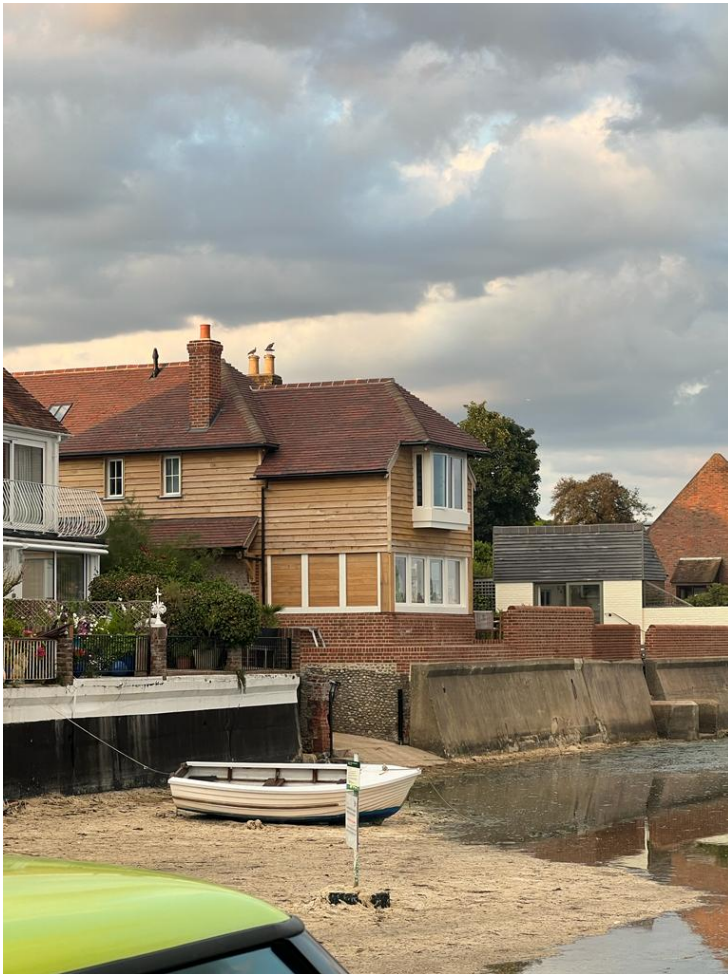
Timber cladding at first floor
