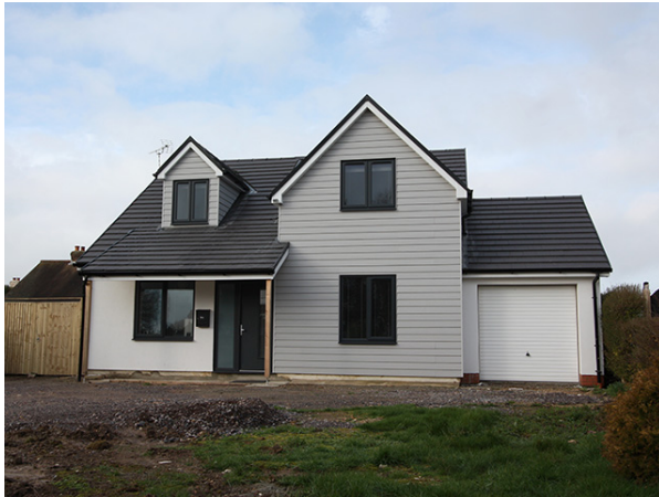
Combination of dark framed PPC aluminium windows & doors, render and composite cladding
