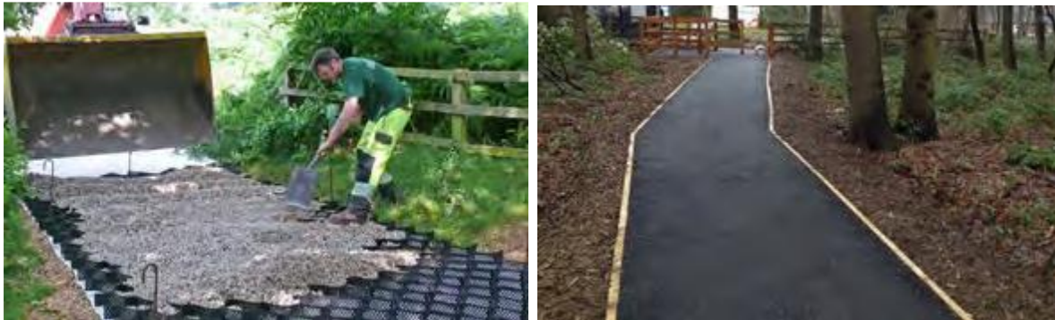
Figure 3.2: Root Protection System Example.
