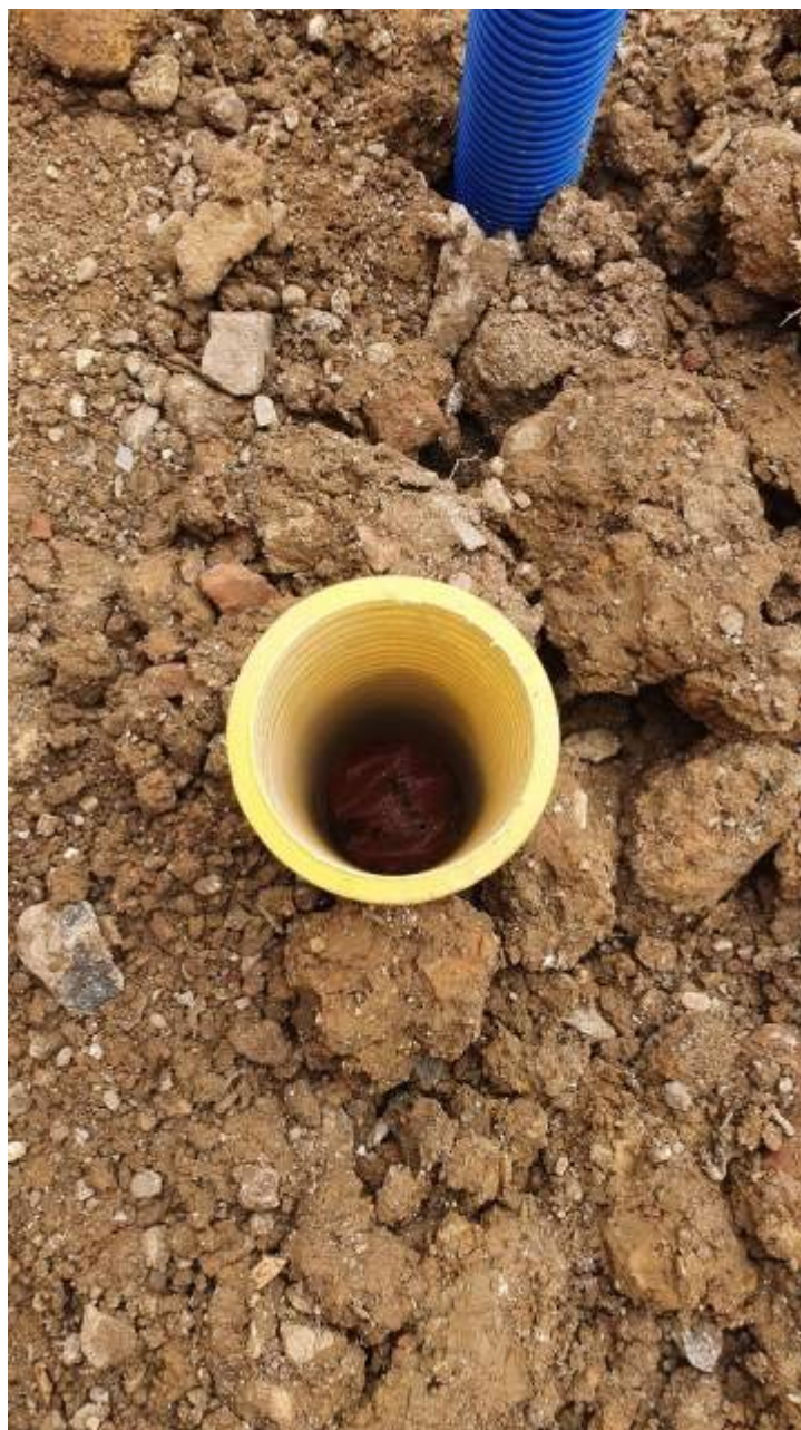
Plate 4 – Orange geotextile beneath subsoil in base of inspection pipe
