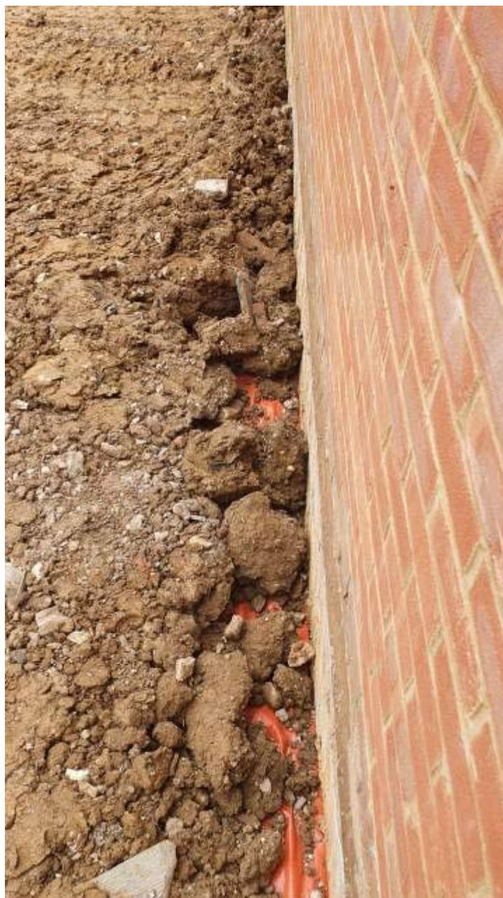
Plate 3 – Orange geotextile membrane visible beneath installed subsoil
