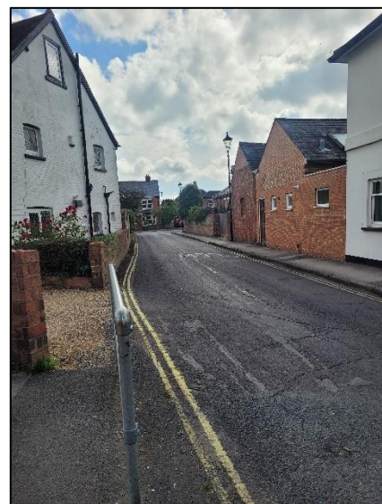
Photograph 5: Existing conditions along Town Hall Road
