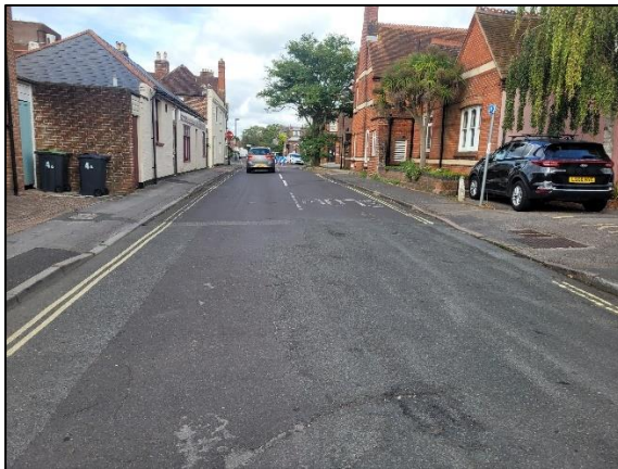
Photograph 4: Existing conditions along Town Hall Road
