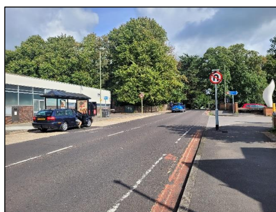
Photograph 2: Existing conditions on East Street
