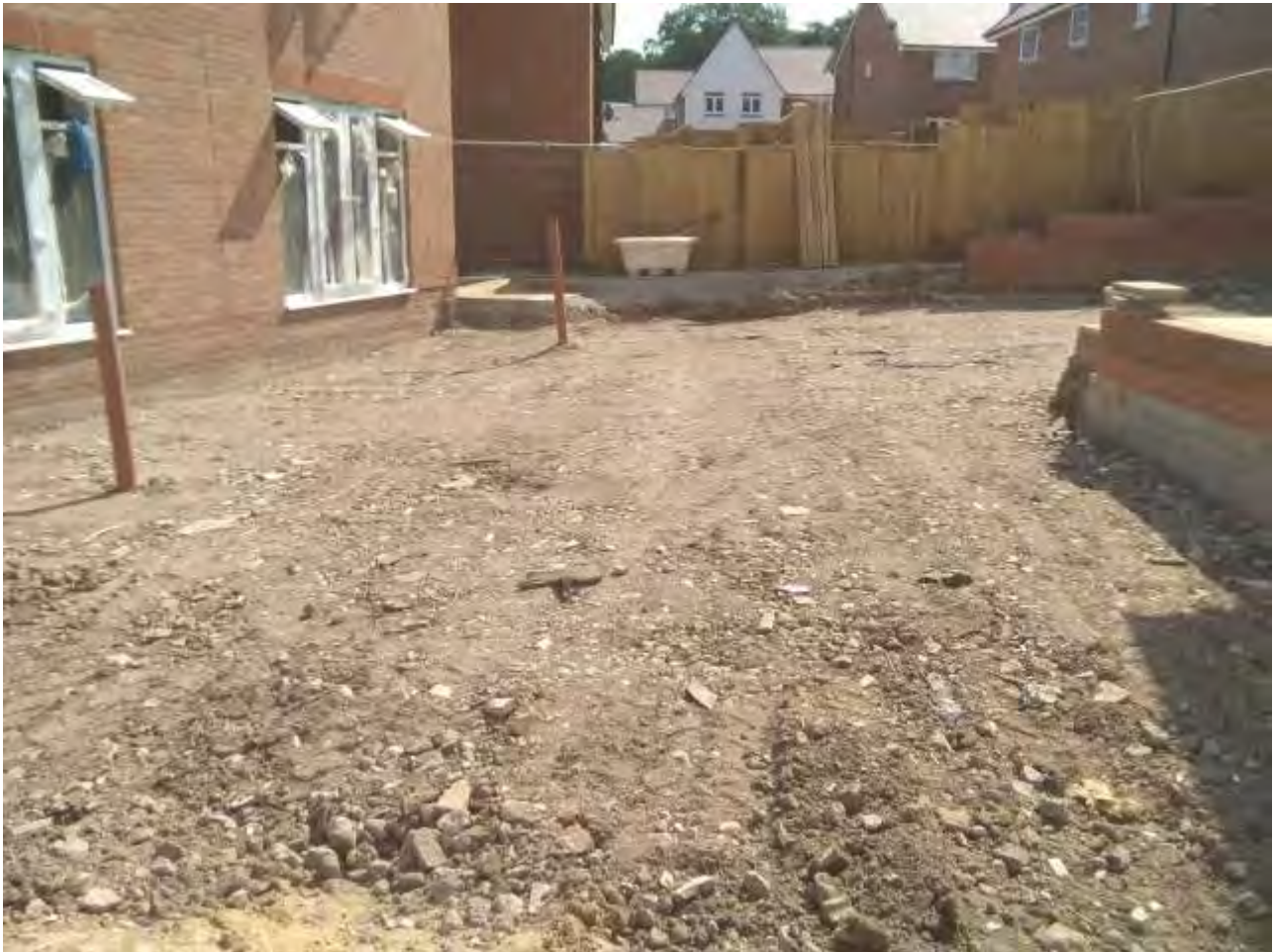
Plate 11 – 21 st July 2021 – view of crushed concrete layer installed across rear of Plots 79-80
