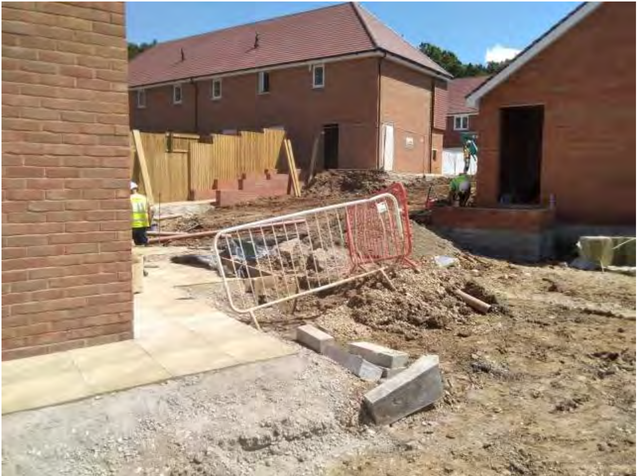
Plate 4 – 9 th July 2021 - view of Plots 79-80 rear garden area prior to reduced dig (the patio was removed in order to undertake reduced dig)
