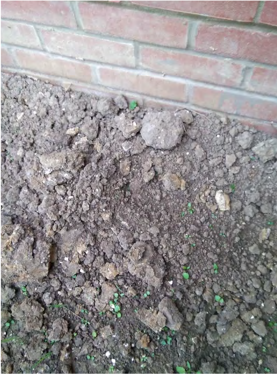
Photo of hole with tape in place
