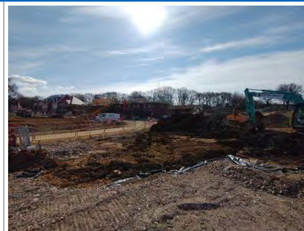
general works area photo
