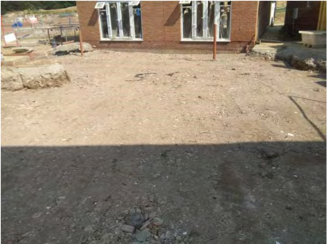
Plate 14 – 21 st July 2021 – view of crushed concrete layer across Plots 79-80
