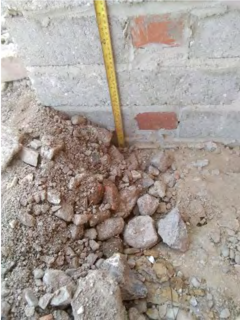
Plate 13 – 21 st July 2021 – view of thickness of crushed concrete layer
