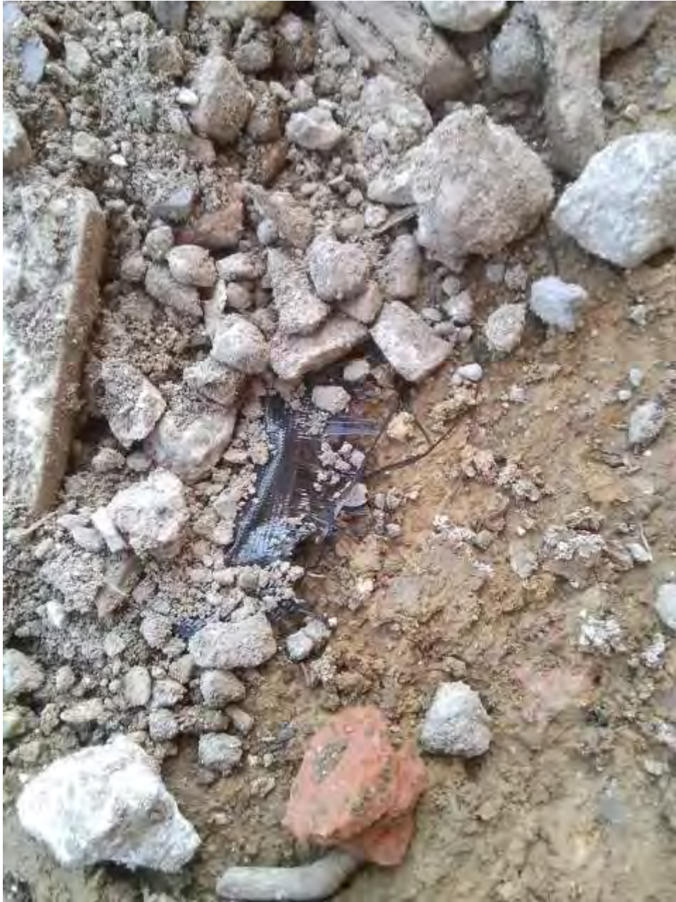
Plate 12 – 21 st July 2021 – view of edge of crushed concrete layer with geo-textile visible
