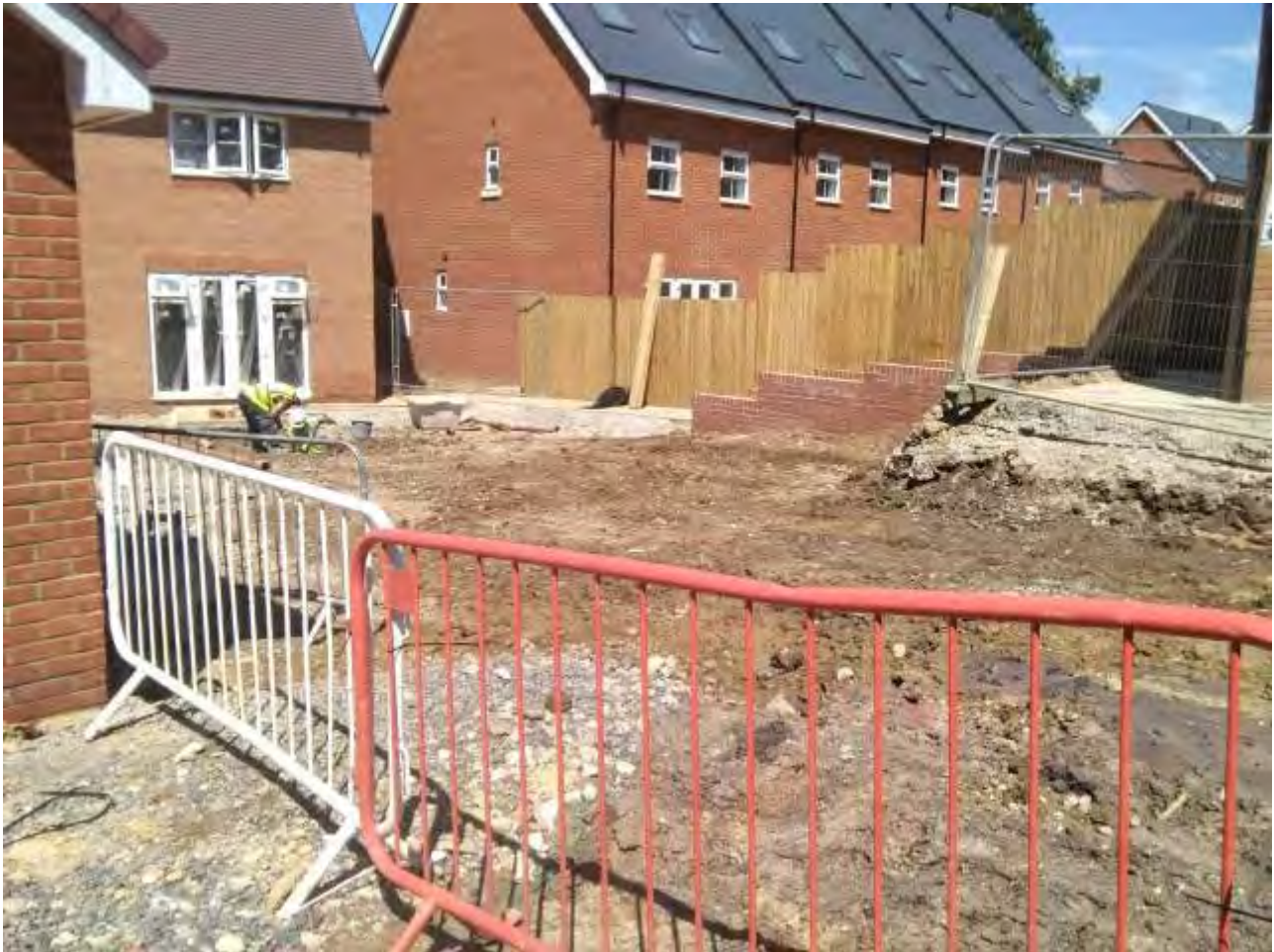
Plate 5 – 9 th July 2021 - view of Plots 79-80 rear garden area prior to reduced dig
