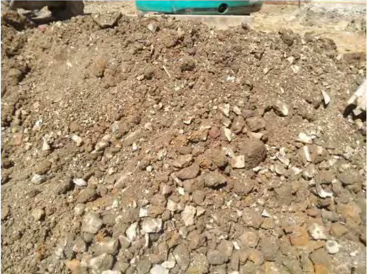
Plate 10 – 19 th July 2021 – excavated material stockpiled for disposal
