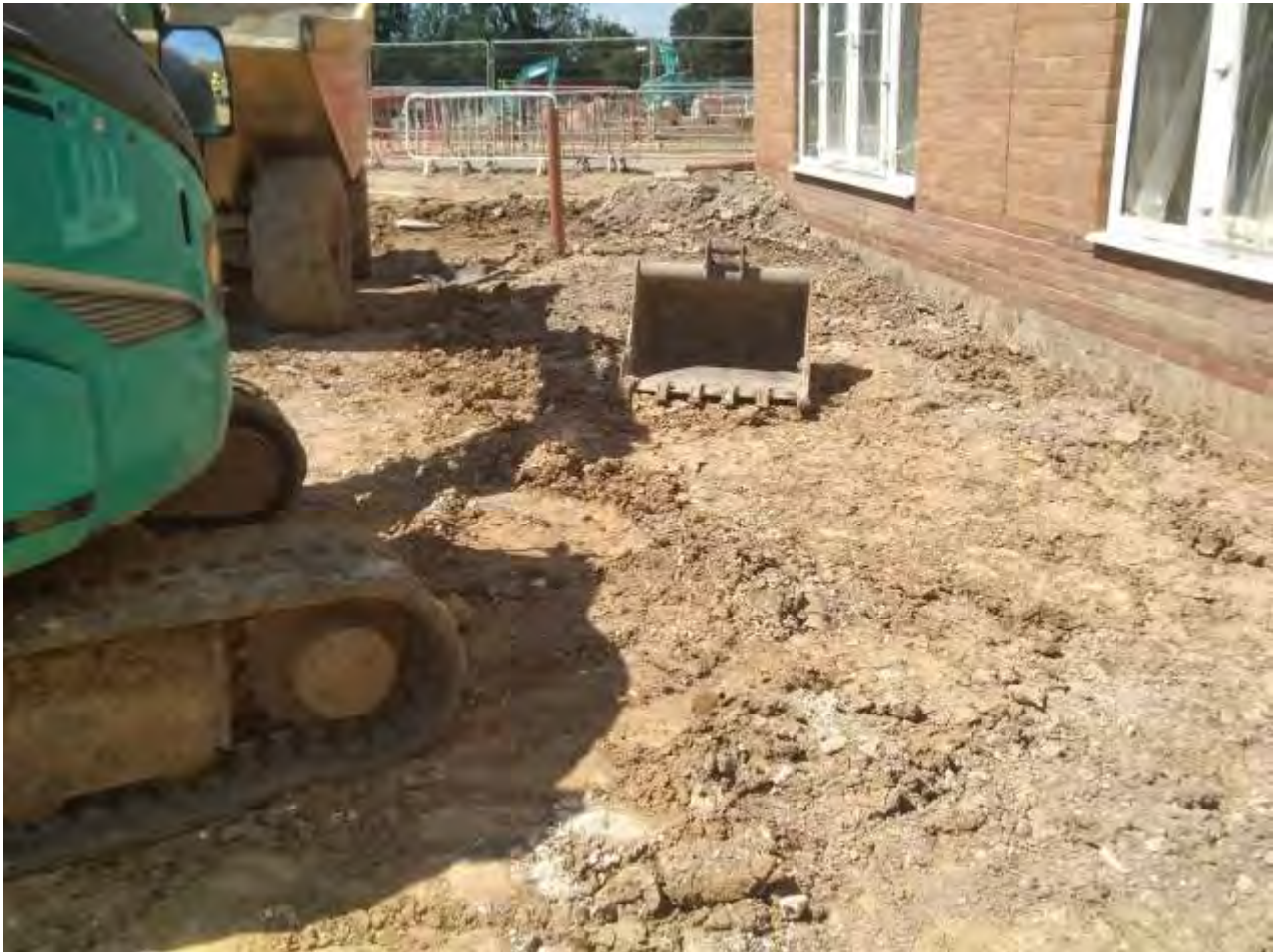
Plate 9 – 19 th July 2021 – reduced dig in rear of Plots 79-80 (previously installed patio removed)
