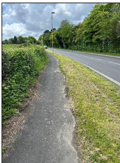
Photograph 4: Existing Conditions along College Road
