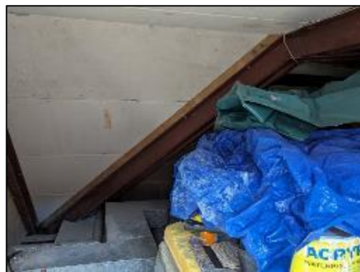
Figure 23: Void being used for storage
