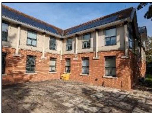
Figure 14: South-eastern elevation of Building B1
