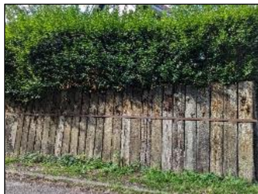
Figure 18: Eastern site boundary sleepers
