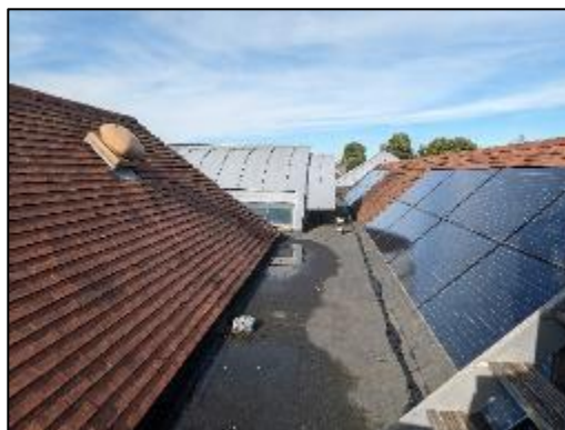
Figure 20: Various constructions on the roof facing west
