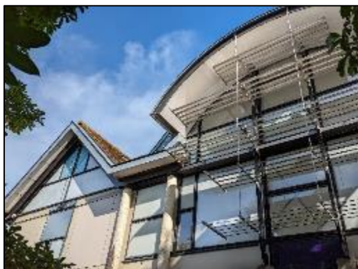
Figure 19: South-western elevation of B1
