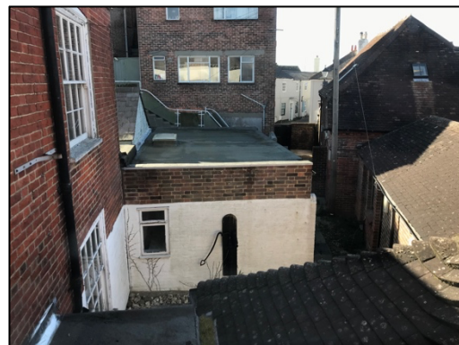
Figure 9 – westernmost flat roof extension
