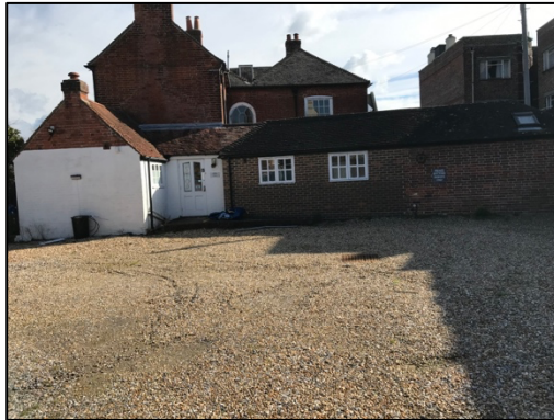
Figure 4 – gravel driveway/parking area in the western section of the site
