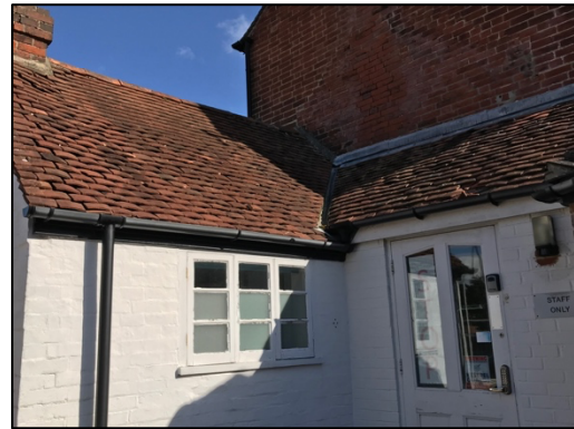
Figure 7 – western gable and mono-pitched extensions
