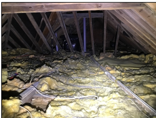
Figure 10 – main roof void
