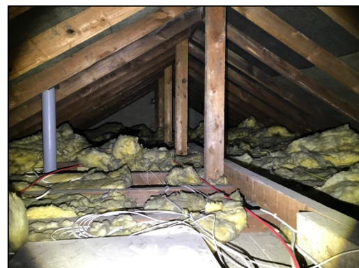
Figure 11 – southern roof void
