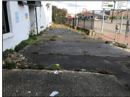
Figure 5 – paved and concrete path in the eastern section of the site
