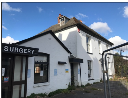
Figure 8 – eastern elevation, with the southern pitched and flat roof extensions
