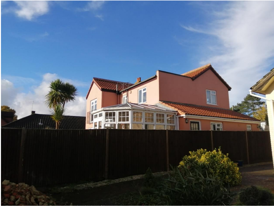
View from garden of 16 Padnell Rd. Here you can see multiple extensions, including a double storey one.
