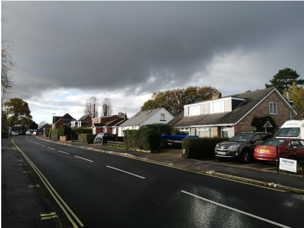
View of No. 5 to 9 Padnell Rd. The architecture is very mixed, and many properties down the road have exploited their loft space with the addition of dormers or are constructed as double storey homes.
