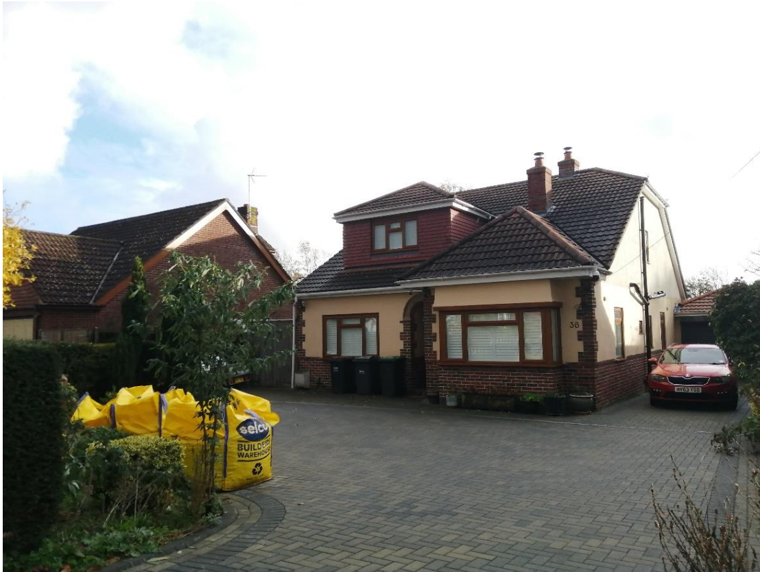
View of No. 36 Padnell Rd.
