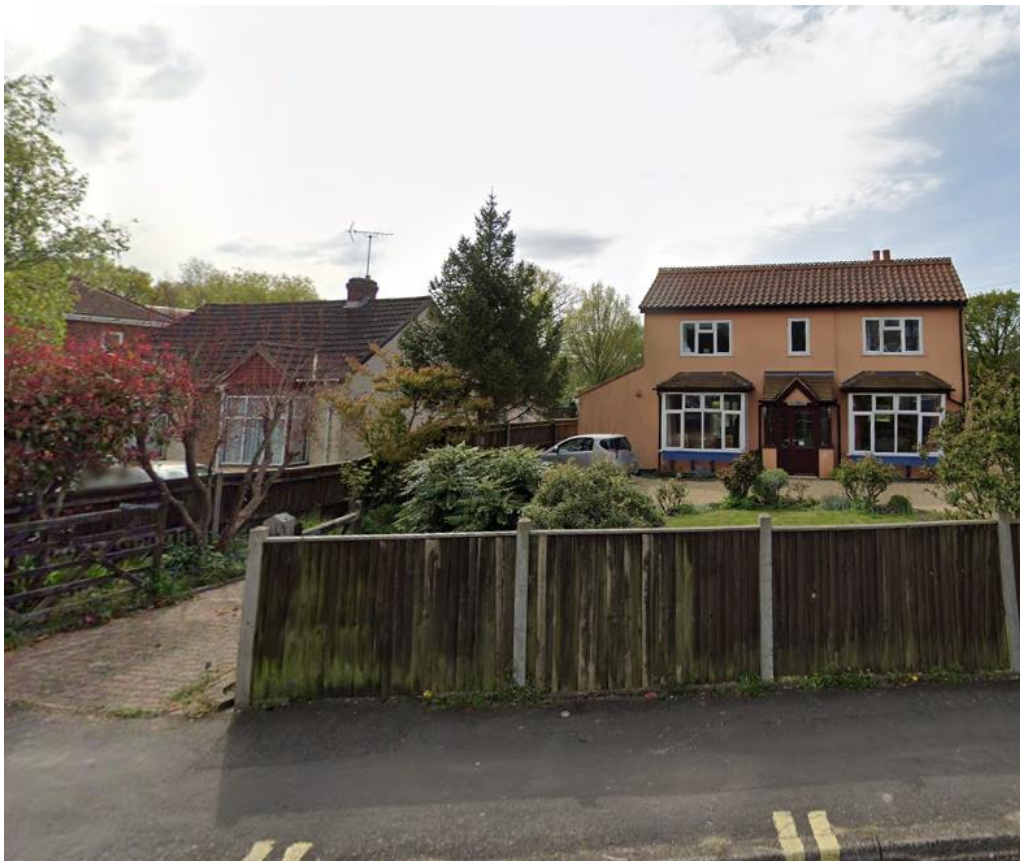
View of No. 16 Padnell Rd. It is 2 storeys so much taller than our property.
