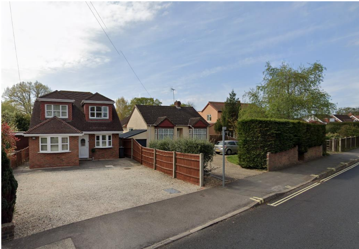
View of No. 20 and 18 Padnell Rd. As you can see our ridge height our property is very low compared to its direct neighbours.
