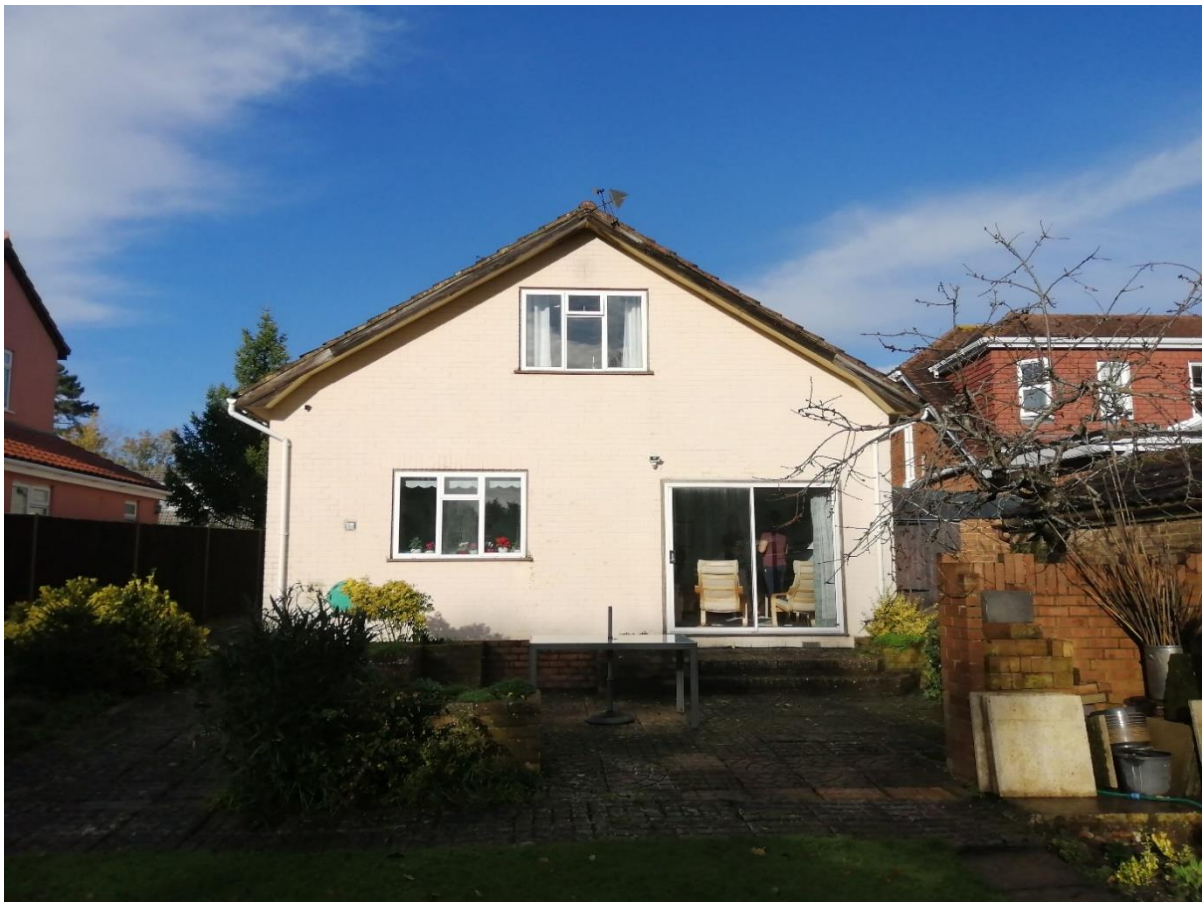
View of rear of house.
