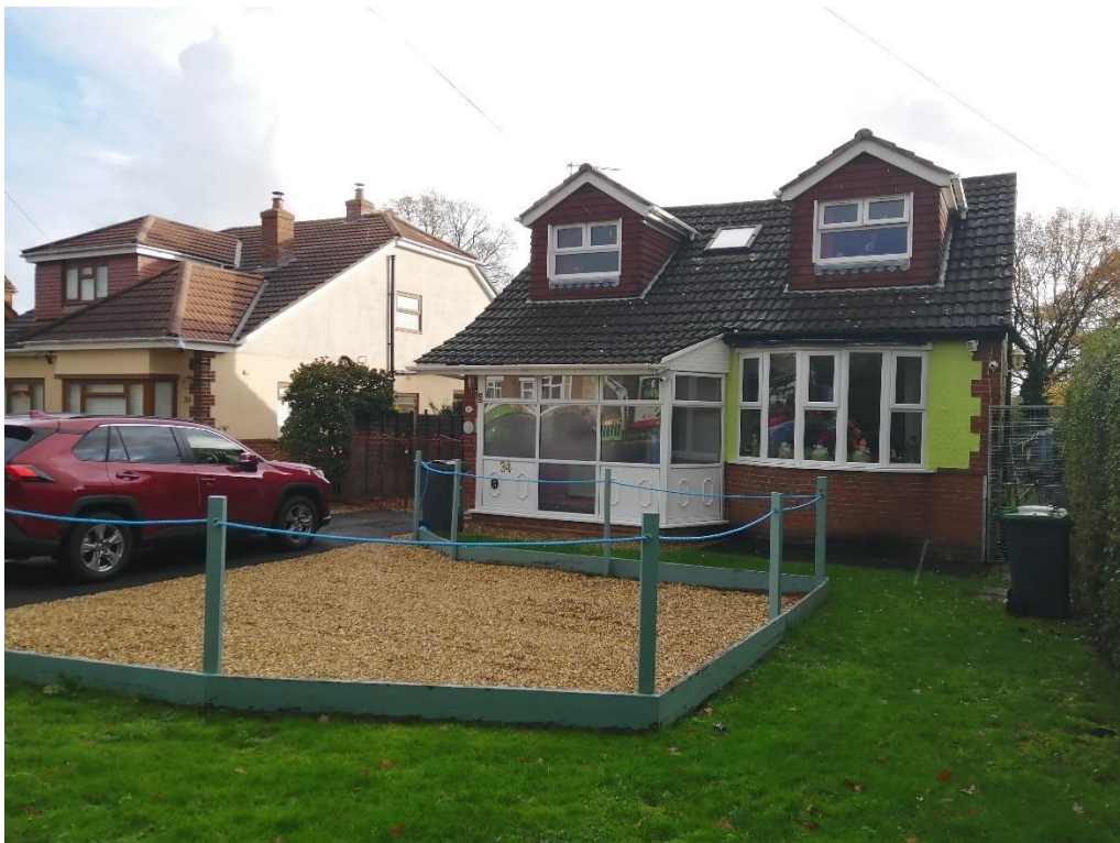
View of No. 34 Padnell Rd.
