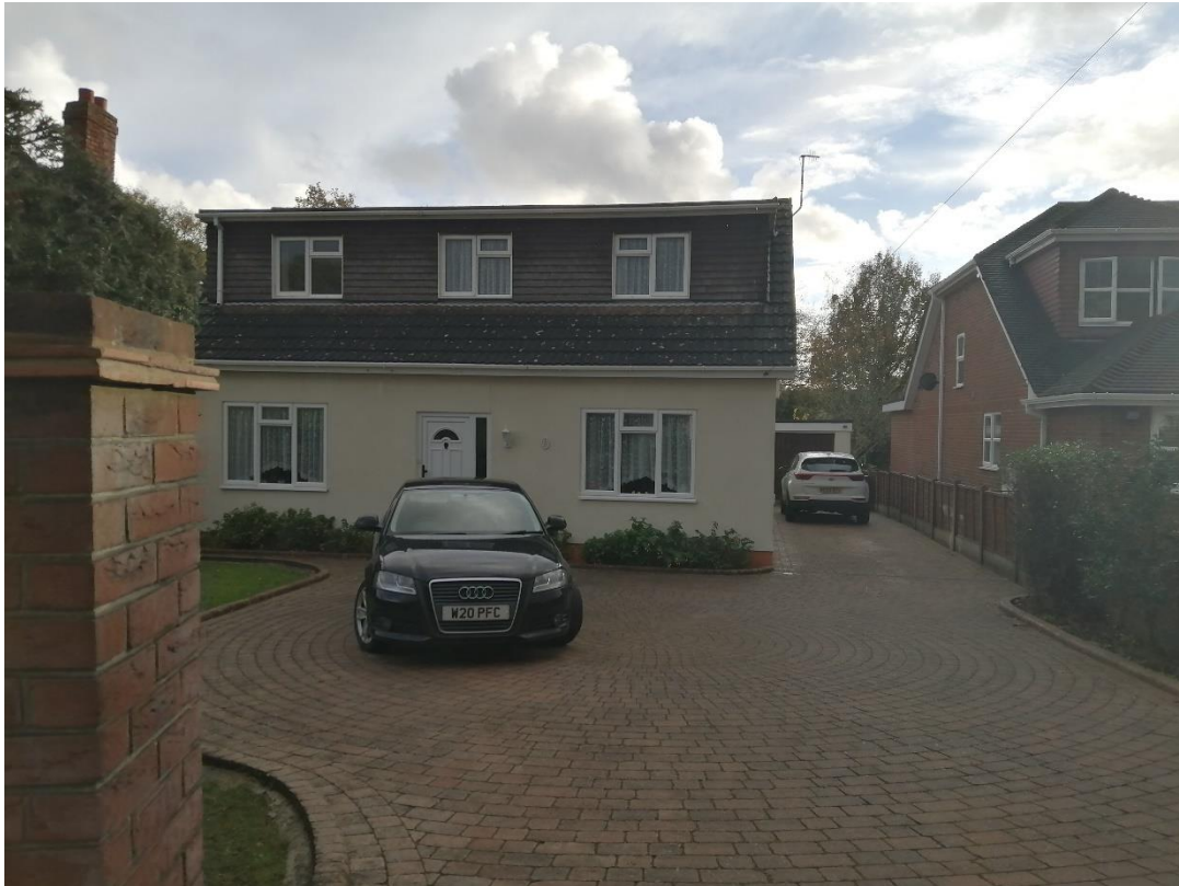
View of No. 22 Padnell Rd. The first floor has been exploited by adding a dormer.
