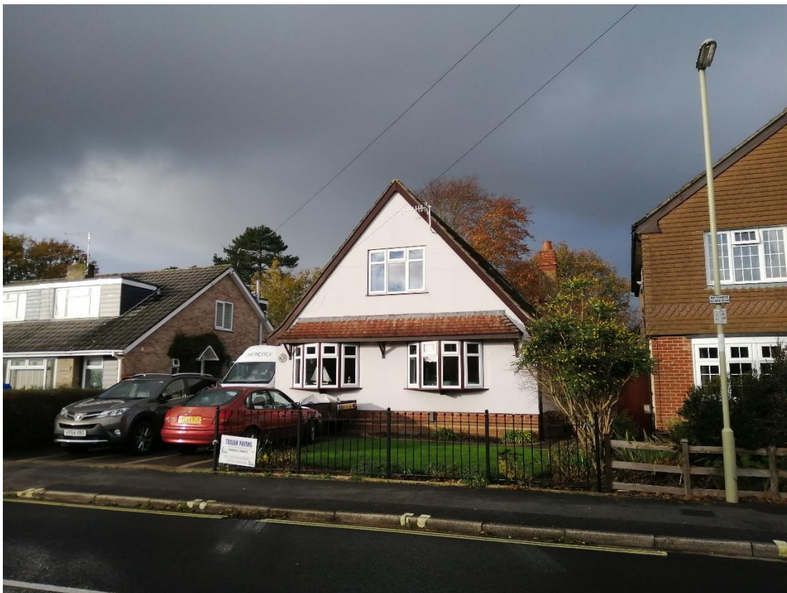
View of No. 9 Padnell Rd.
