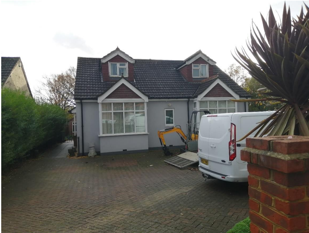
View of No. 26 Padnell Rd. Again, this has been exploited with dormers thus increasing the useability of the roof space.
