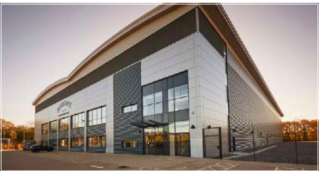
7 Close up view of existing Fat Face build
